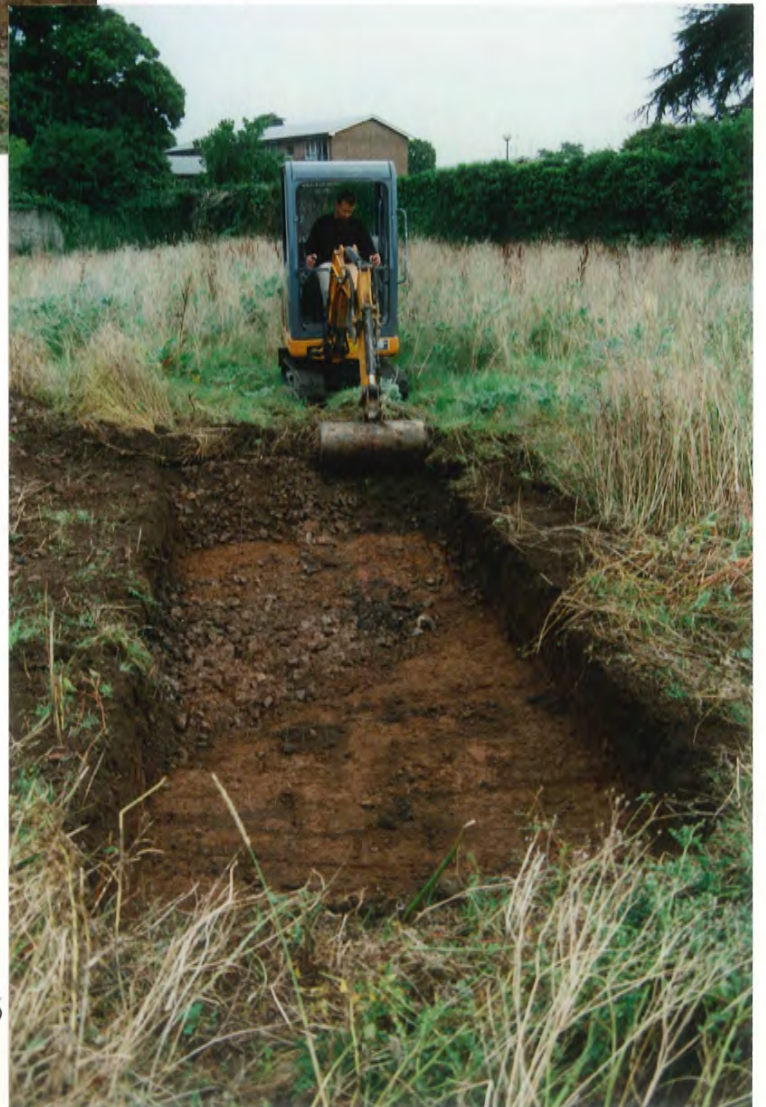
→Plate 10 Mini excavator at work in Trench 6
