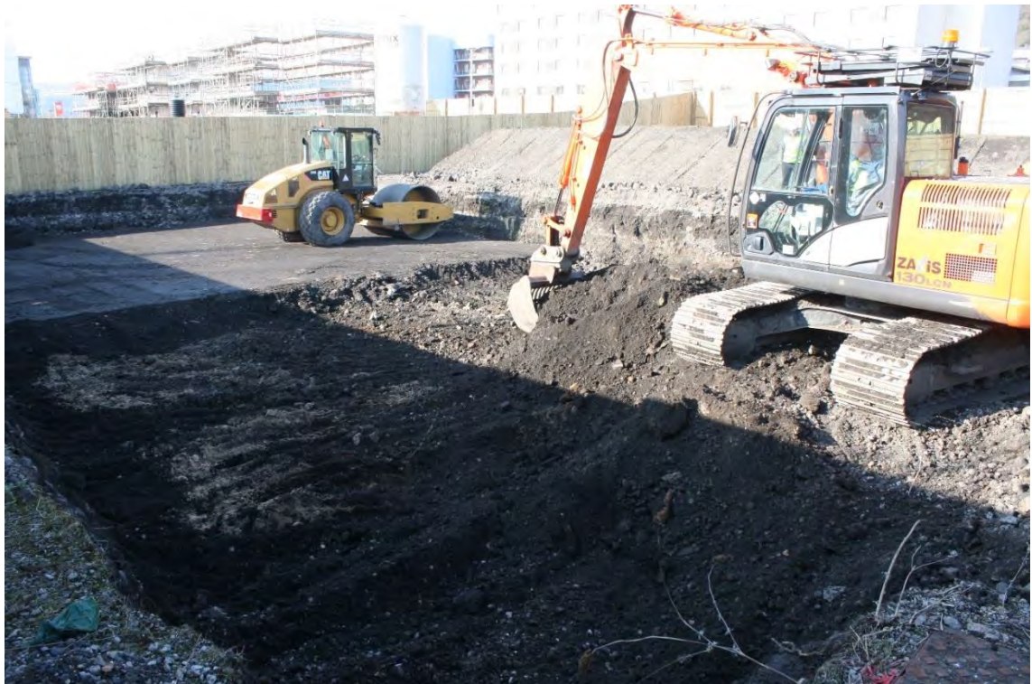
Plate 10: View northwest of western half of plot 6-11 being backfilled and compressed.
