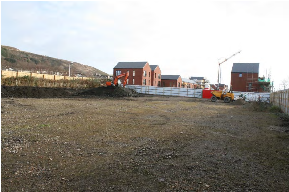
Plate 1: View east across the site prior to excavation works.
