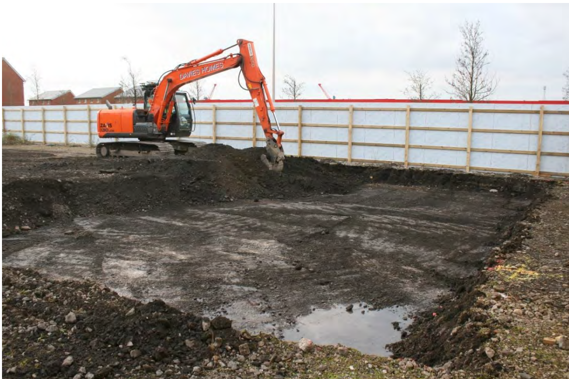
Plate 4: View southeast of initial excavation of plot 6-11, through deposits 003, 002 & 001.
