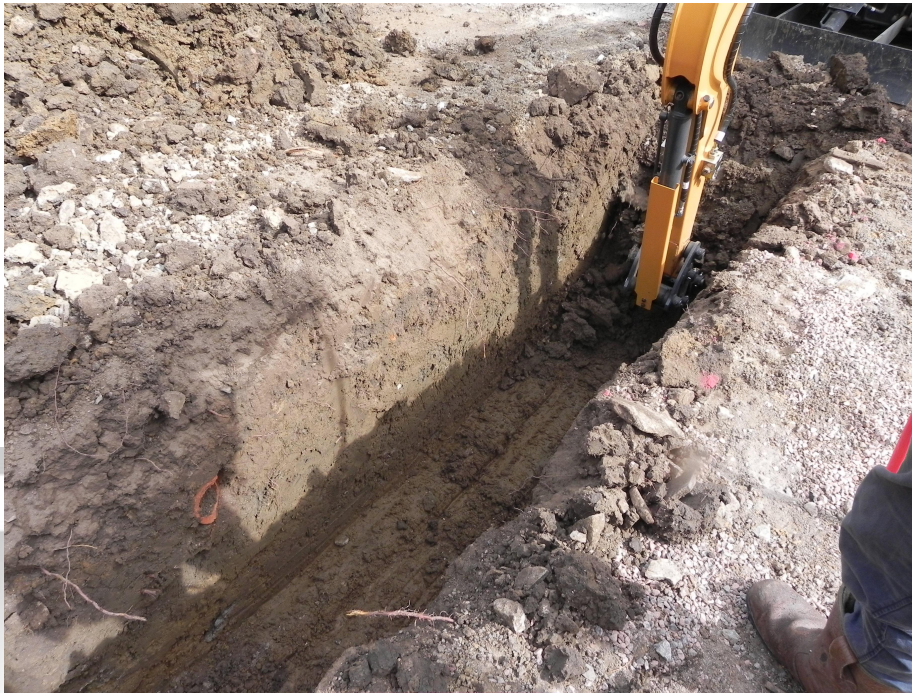
Figure 5 Trench A, being excavated down to level: 1,100mm
