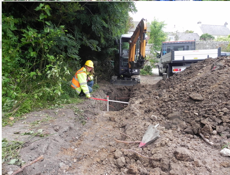
Trench C active recording looking north
