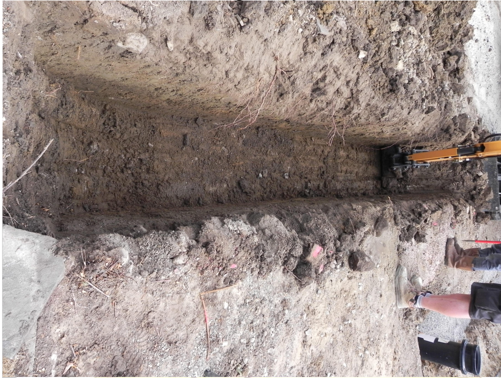
Figure 13, excavation of trench A
