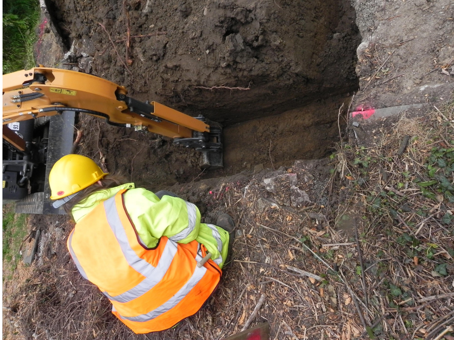
Figure 15, inspecting trench B
