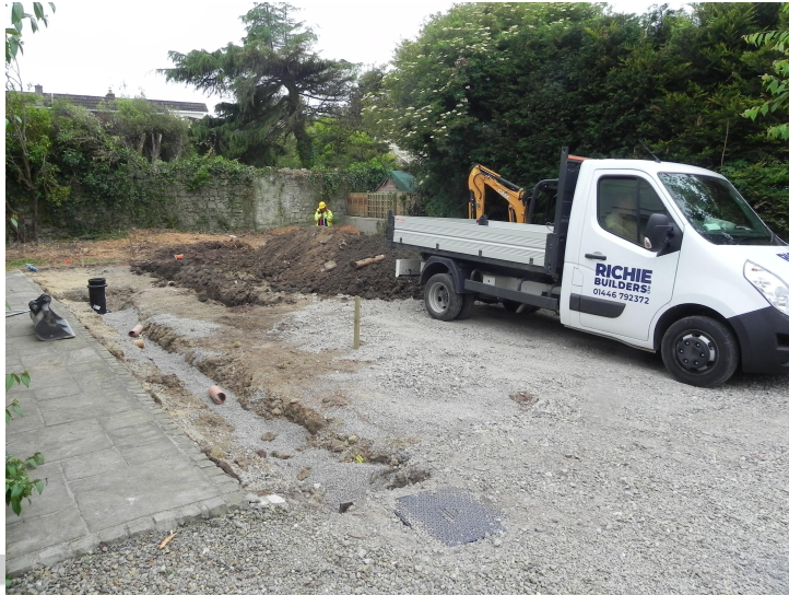
Figure 7, Richie Builders on site
