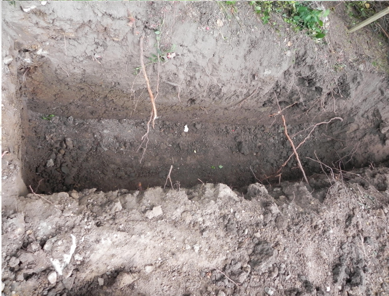
Levels in trench C
