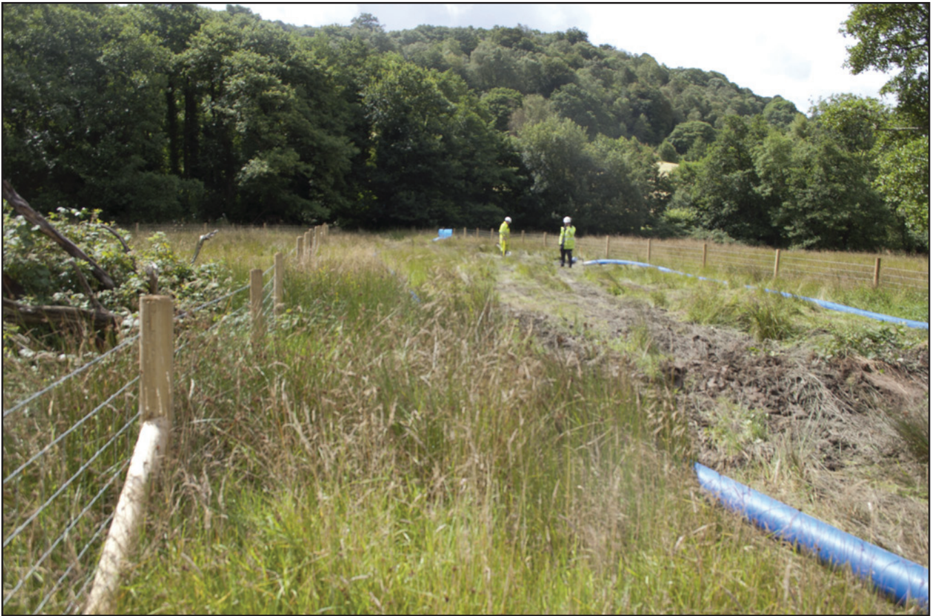
Plate 01: General view looking south along pipeline easement route (archive image: G2528_010).
