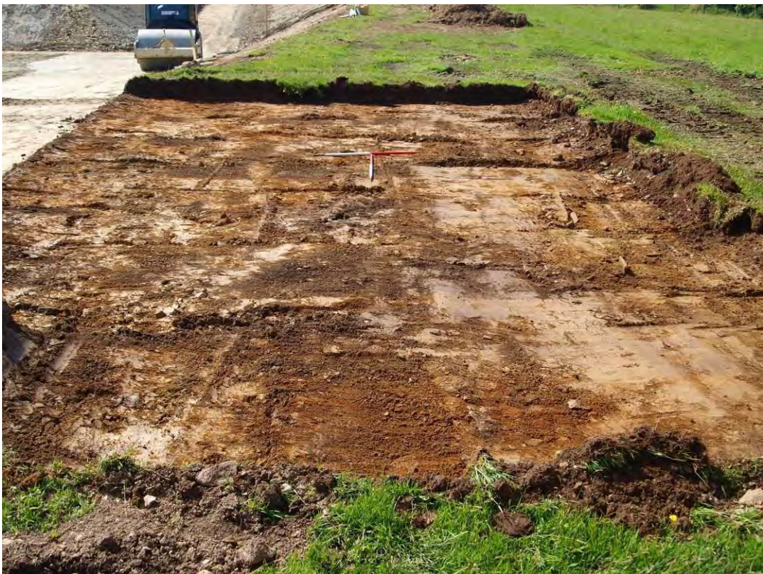
Photo 8: View south across the area stripped for the substation. 1m scales.
