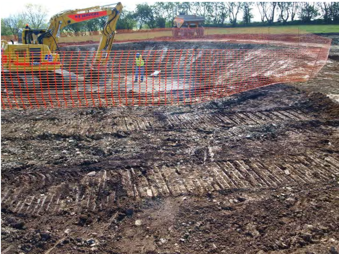
Photo 6: View southeast across the excavated area of the wind turbine foundations.
