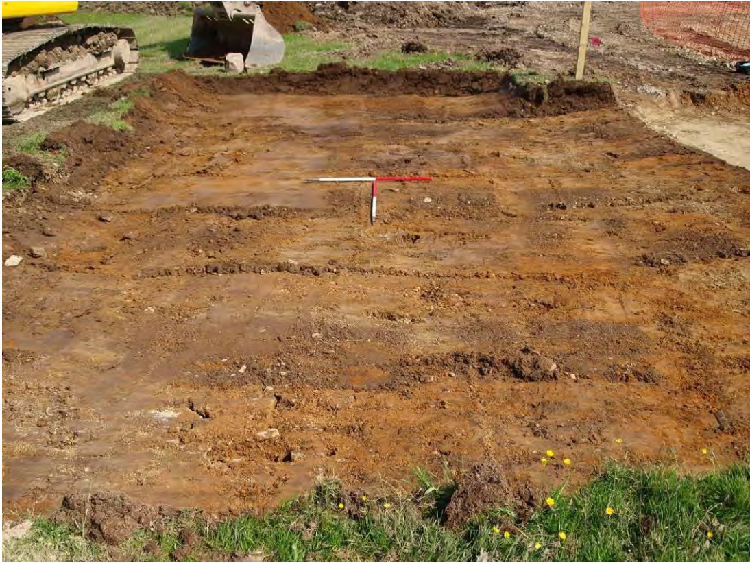
Photo 7: View north across the area stripped for the substation. 1m scales.
