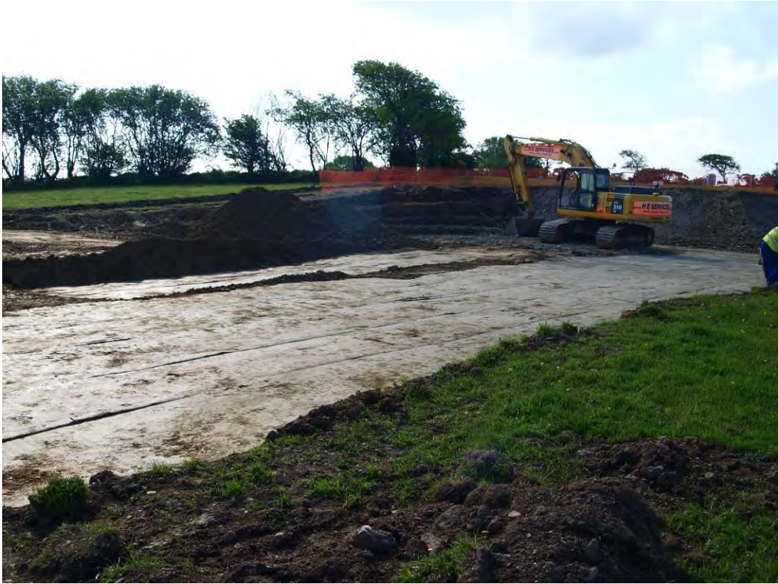
Photo 5: View southeast across the crane pad foundation area.
