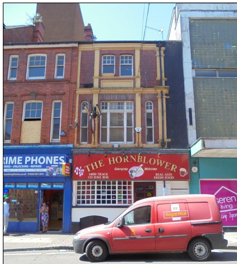
Photo 2: The eastern facade of no.126 Commercial Street
