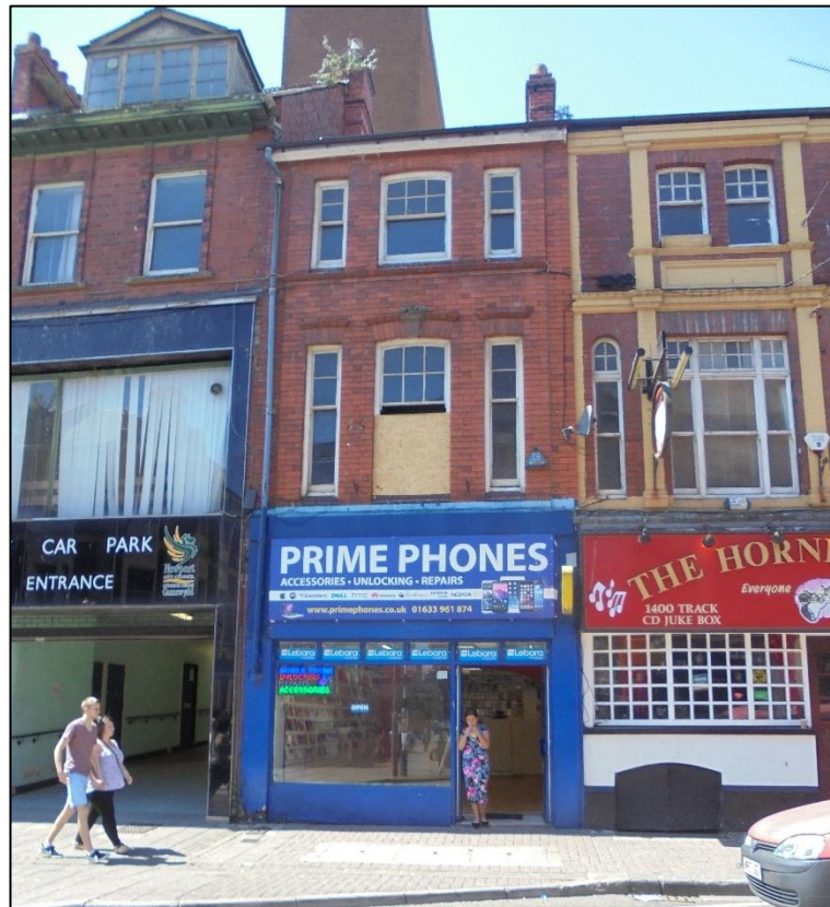
Photo 3: The eastern facade of no.125 Commercial Street
