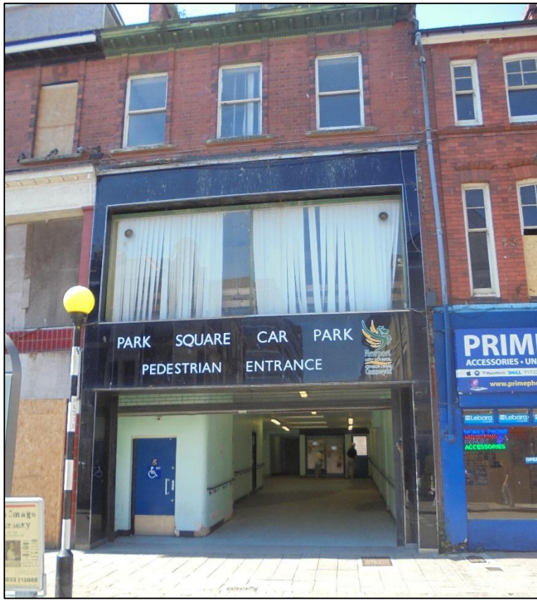
Photo 4: The eastern facade of no.124 Commercial Street
