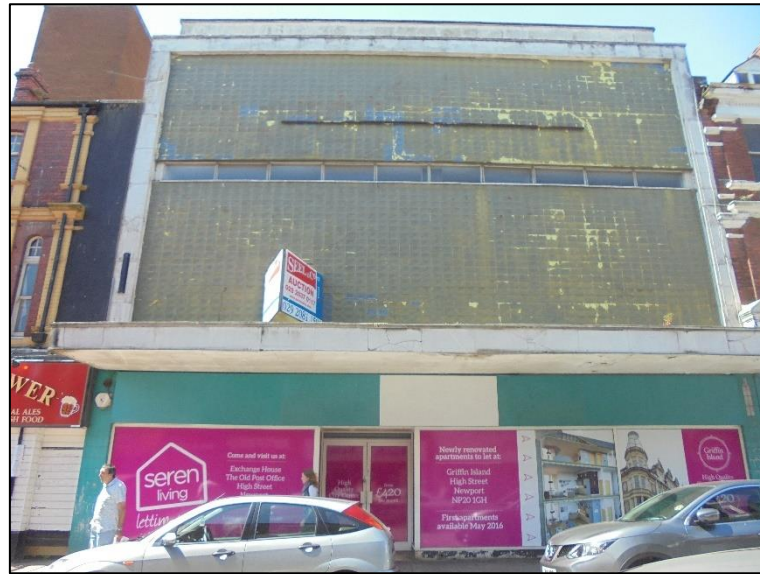
Photo 1: The eastern facade of no. 127-129 Commercial Street
