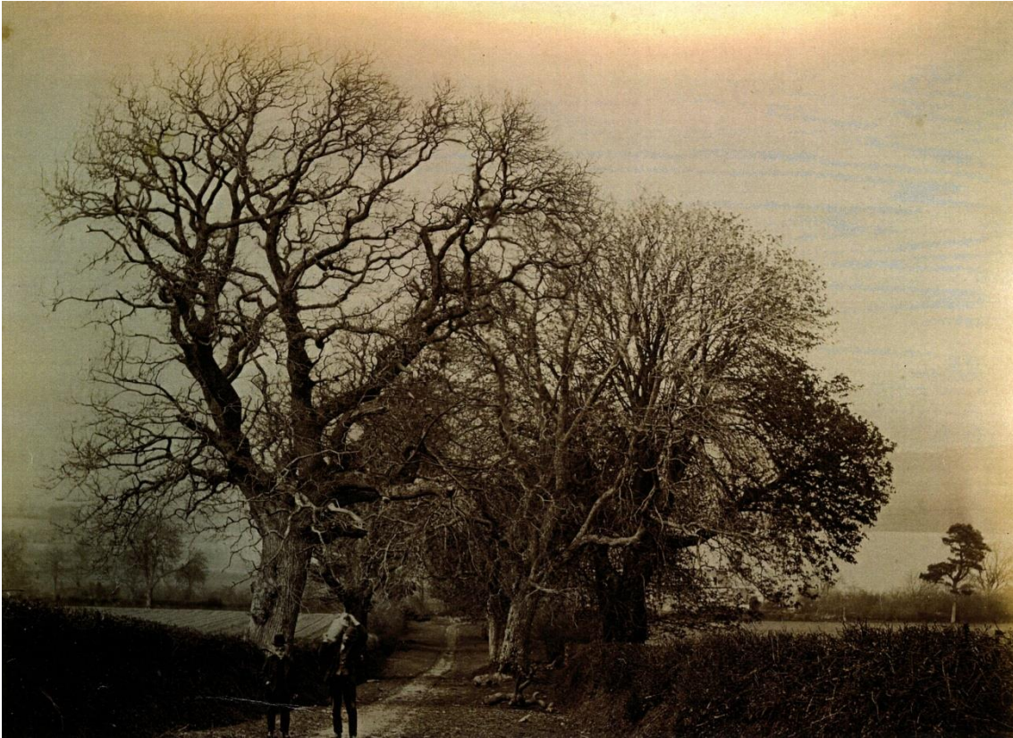
Figure 9: The drive and avenue to the house probably in 1870. © National Library of Wales, Crawshay Album / NLW 565 W6
