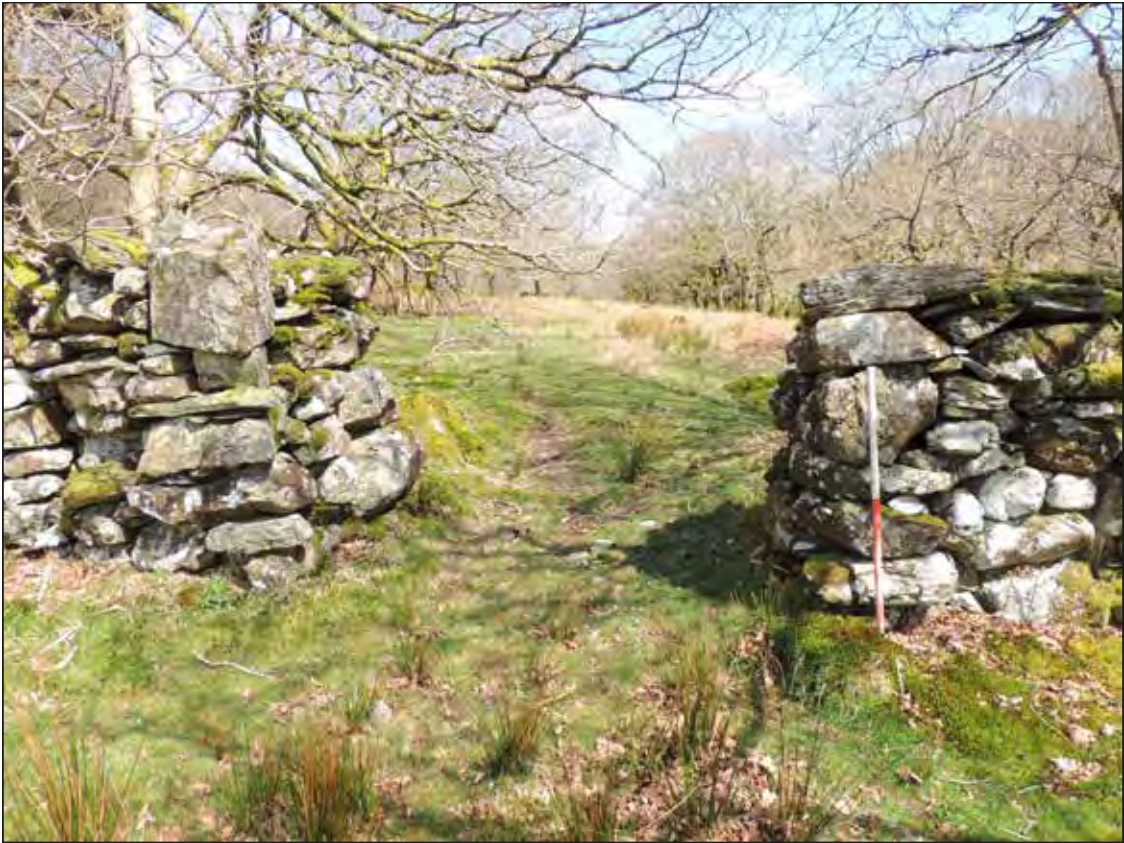
Plate 13. Penstock route c. SH62445 44123. Looking NE.
