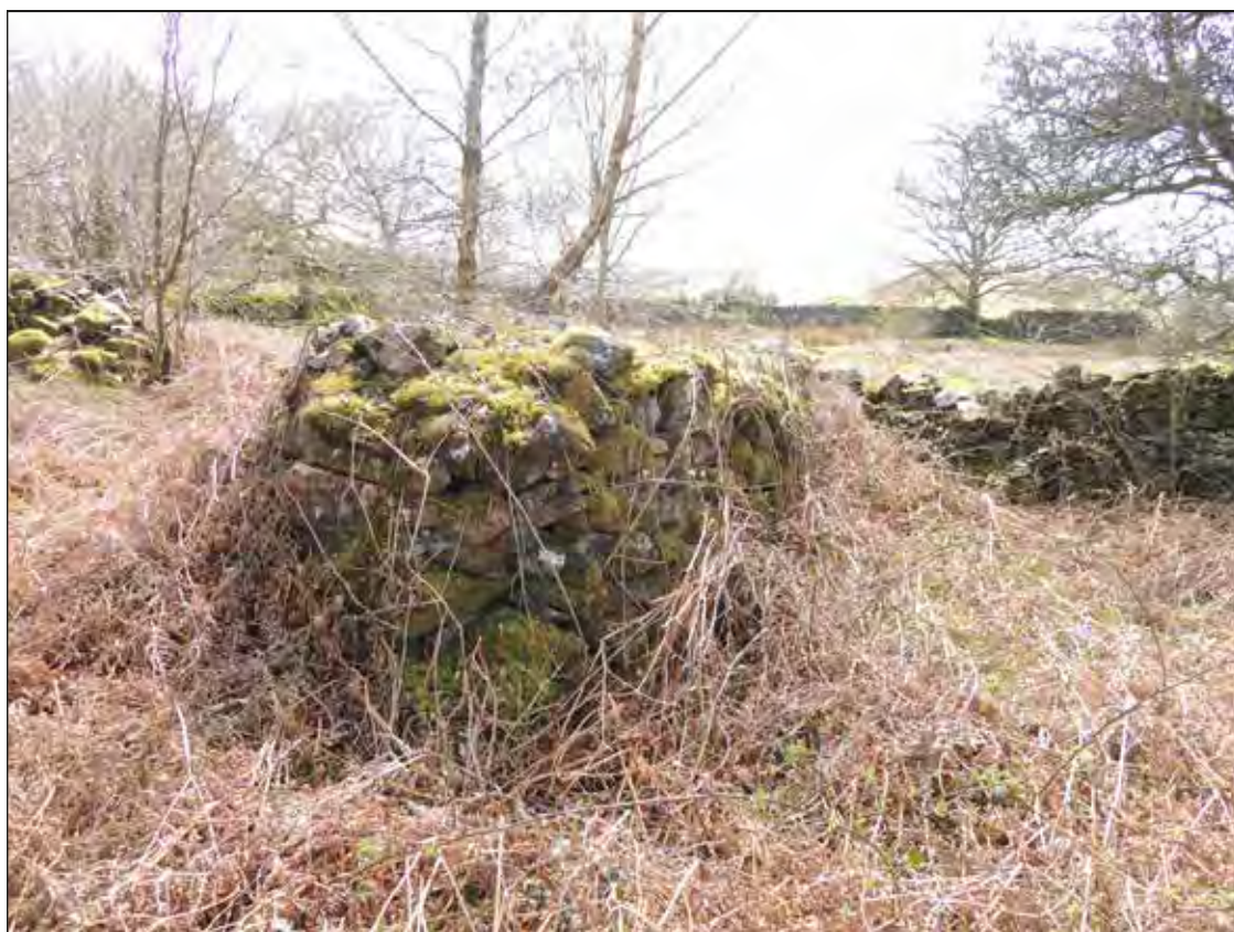
Plate 32. Remains of dry-stone wall recorded in OS historical maps. Looking S.
