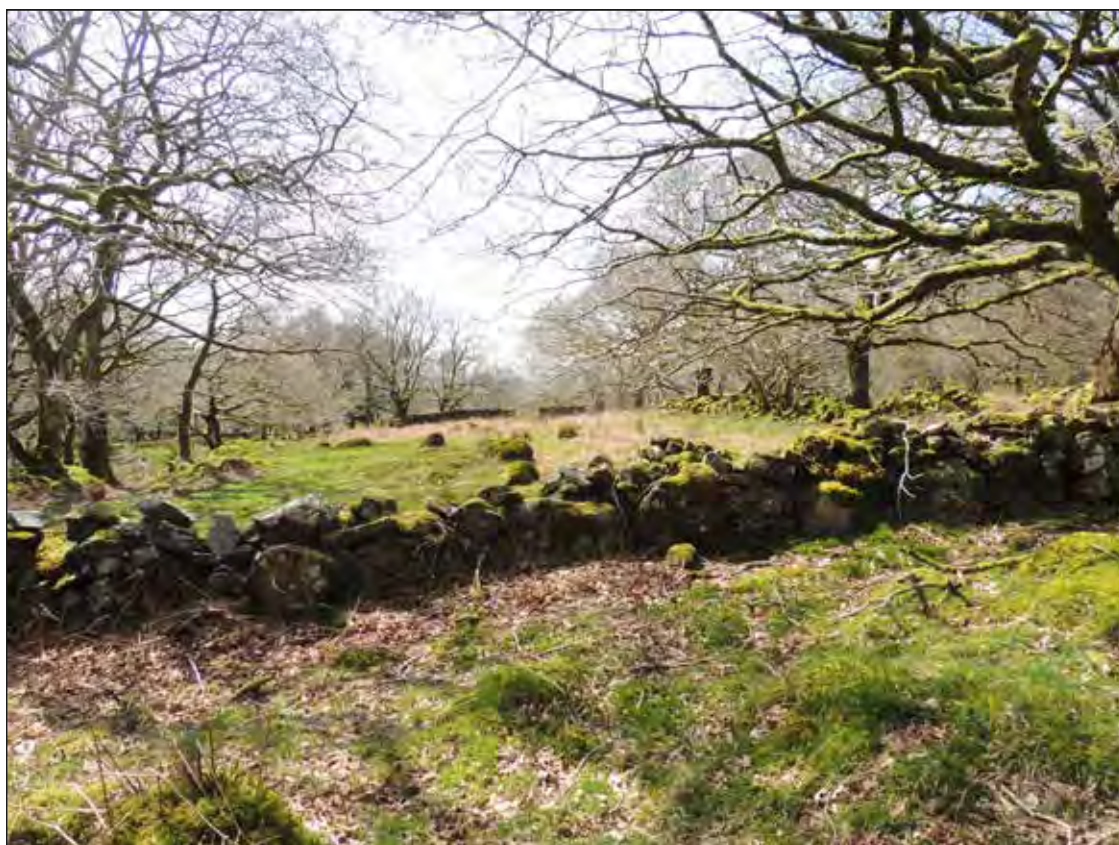
Plate 11. View of penstock route c. SH62501 44165. The route will cut through the dry -stone wall shown.
