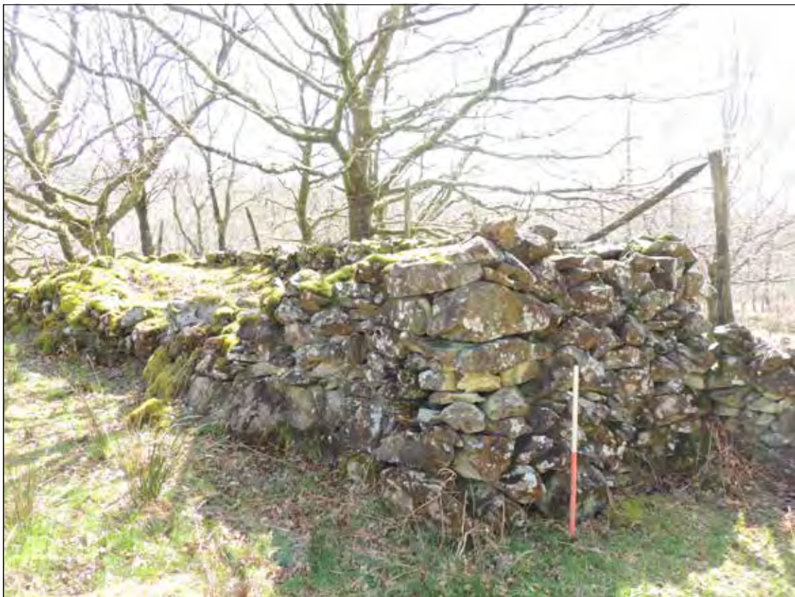
Plate 18. Remains of structure, possible sheep fold. Oblique view.
