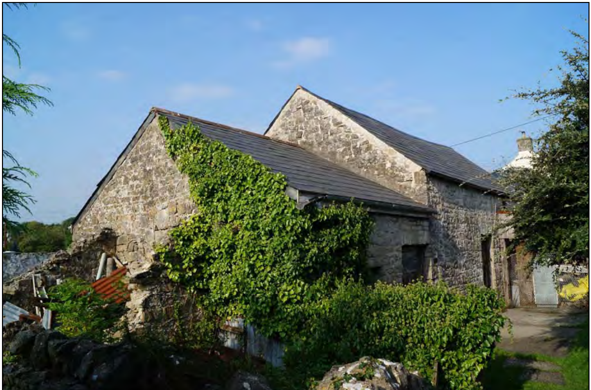
Plate 4: RCT2017_104, The western end of the building, showing the western ruined pigsty (C) and its yard (D), the low western extension (B) and the main barn (A), looking northeast.
