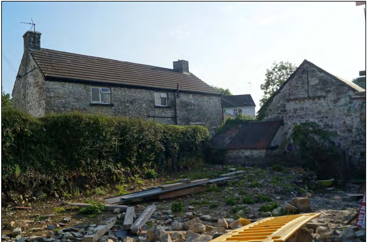
Plate 14: RCT2017_114, Rawley Court house with the barn (A) to the right of the photograph, looking south southwest.
