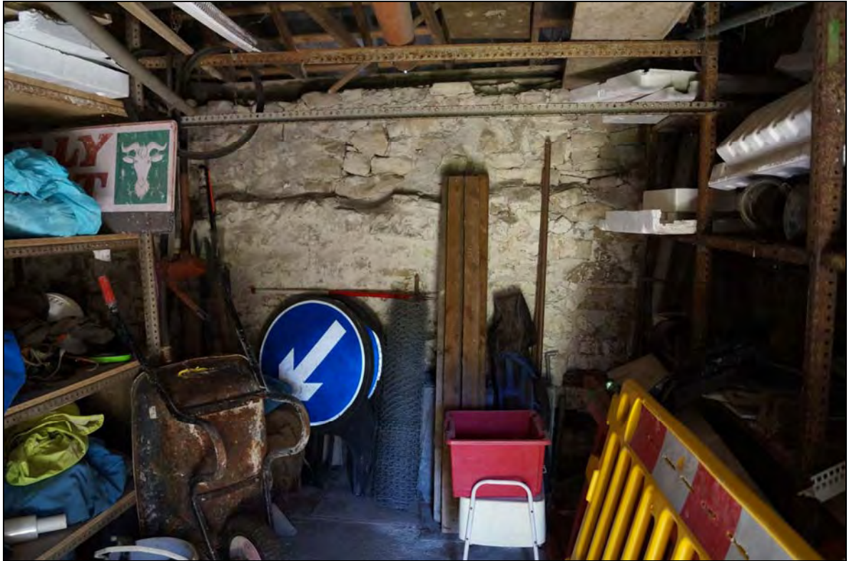
Plate 27: RCT2017_127, Internal view of northern wall of extension (B), looking north-northwest.
