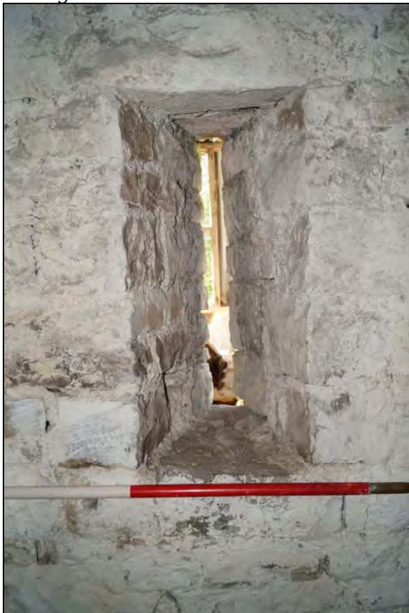
Plate 20: RCT2017_120, Internal view of ventilation slit in southern wall of barn (A), looking south southeast.
