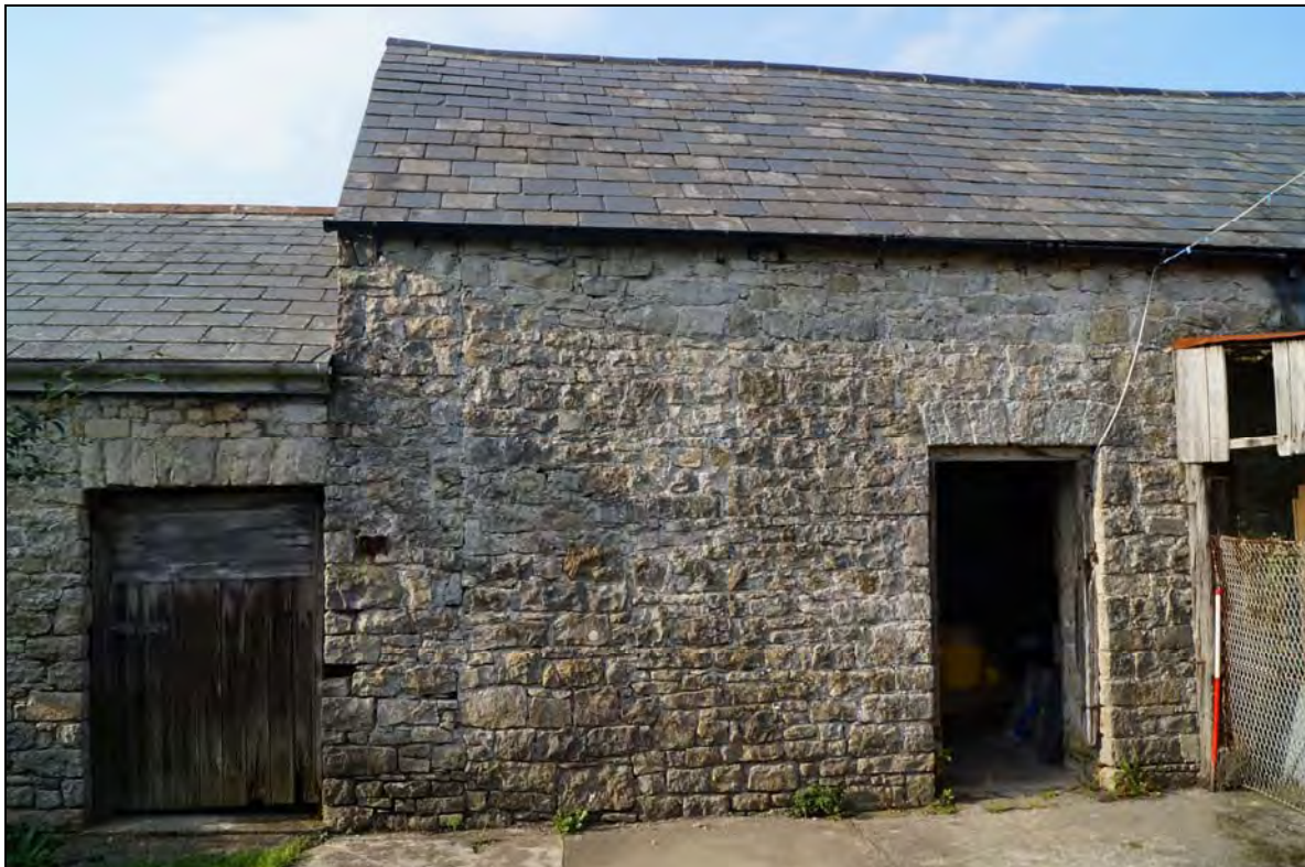
Plate 2: RCT2017_102, The western end of the main barn (A) showing join and difference in roof height with (B) to the west (left), looking north northwest.
