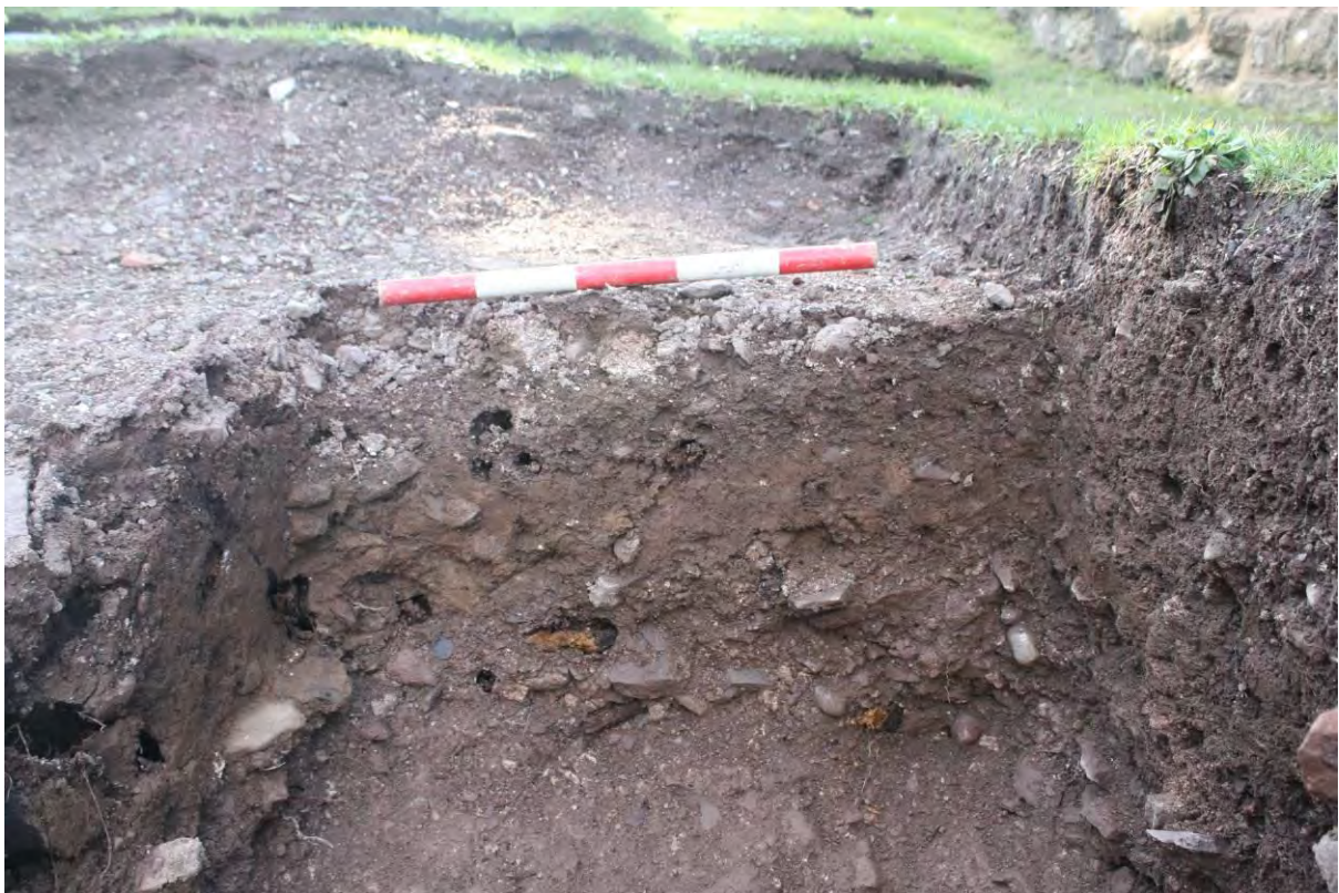
Photo 10: South facing shot of the southern section of the excavated slot within the evaluation trench. 0.5m scale.
