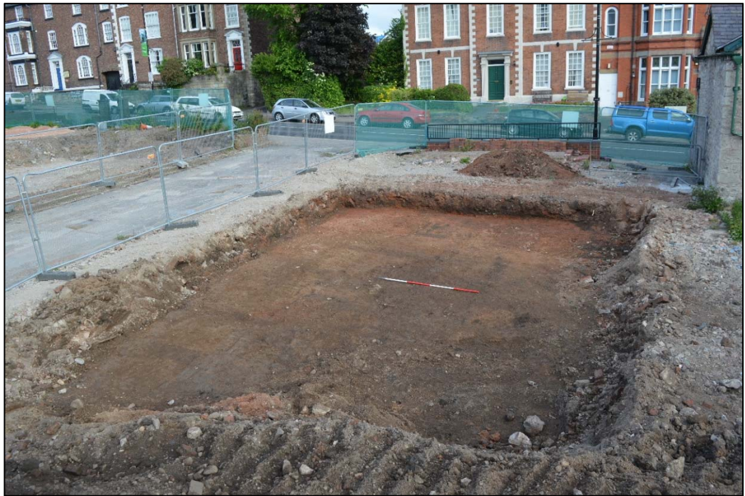
Fig. 6. Overview of the linear features in the western and northern area of the site, truncated by a large pit and later disturbance in the centre of the area. CPAT Photo 4030-0020
