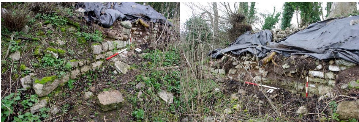
Figure 38: Trench 10 wall [167] in 2017
