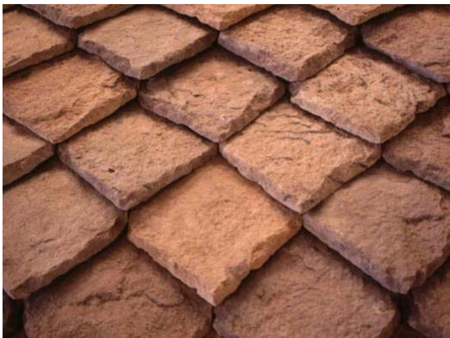
Figure 73: Reconstruction of stone slates from Brading Roman Villa (Isle of Wight). Image Simon I Hill, Oglander Roman Trust
