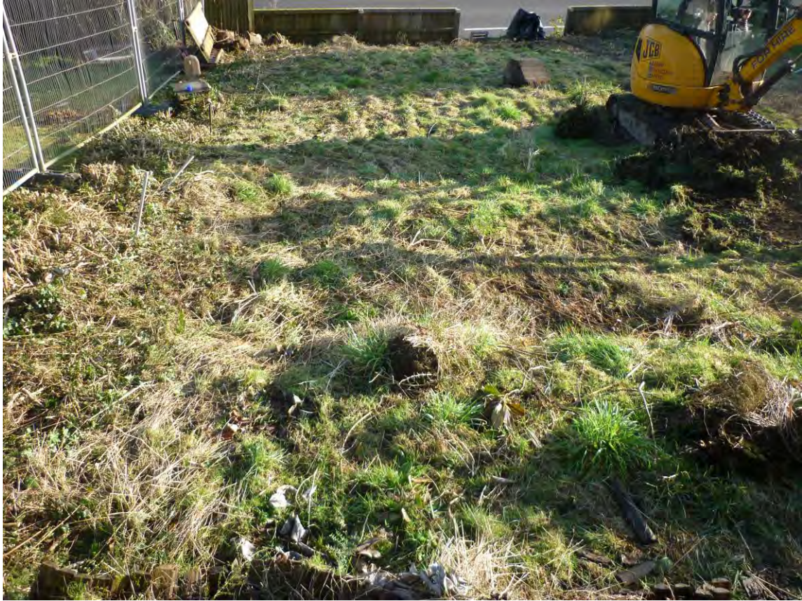
Plate 13: Working shot, 8T excavator removing topsoil
