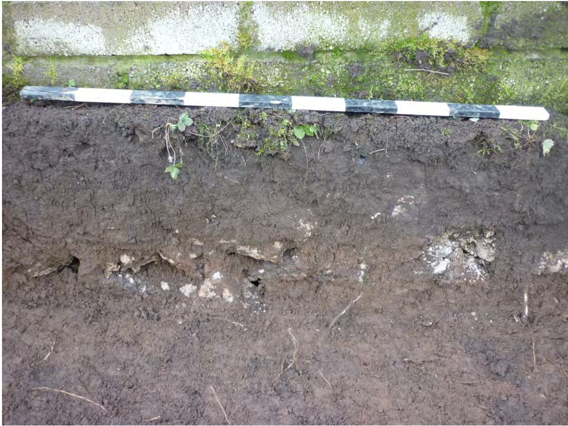
Plate 15: Retaining wall, close up.
