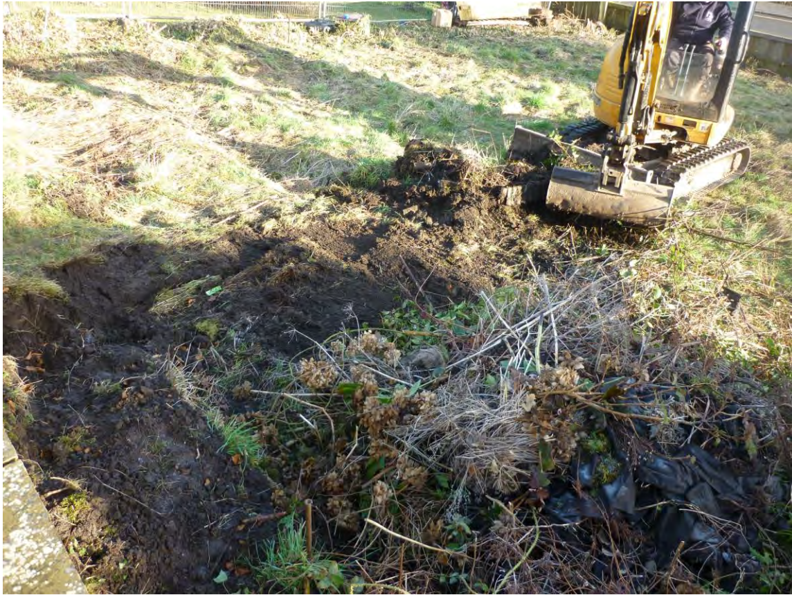
Plate 11: Working shot, 8T excavator removing topsoil
