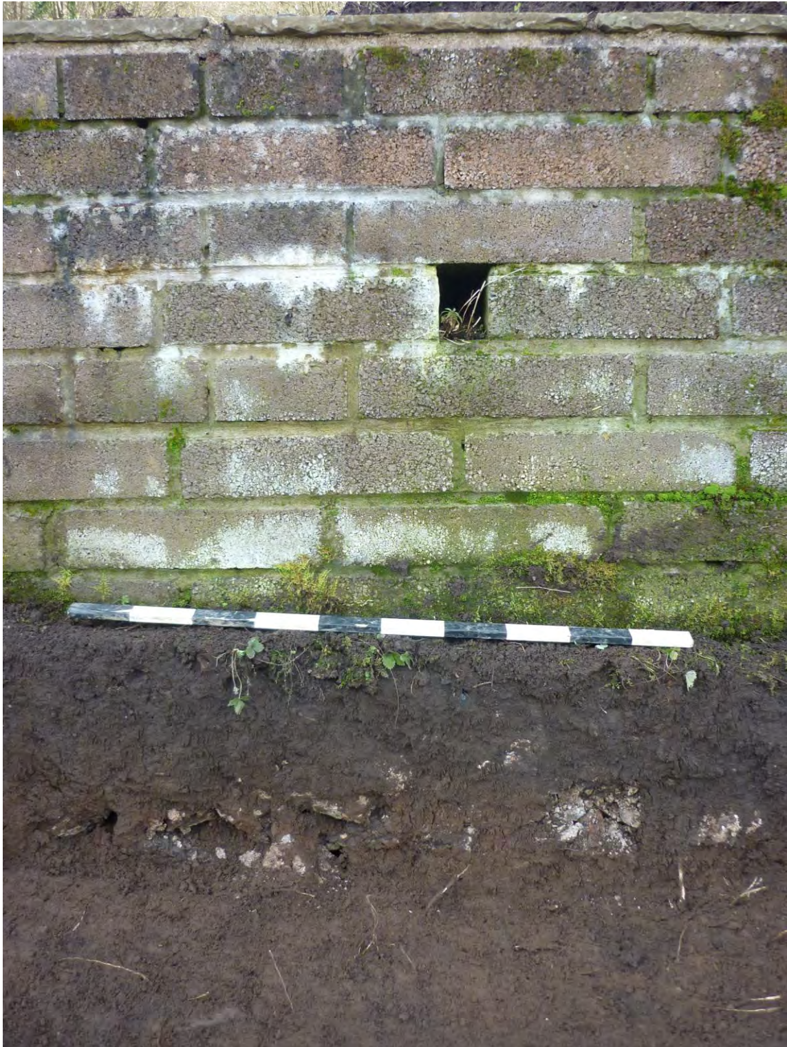
Plate 14: Retaining wall at the southeastern side of site
