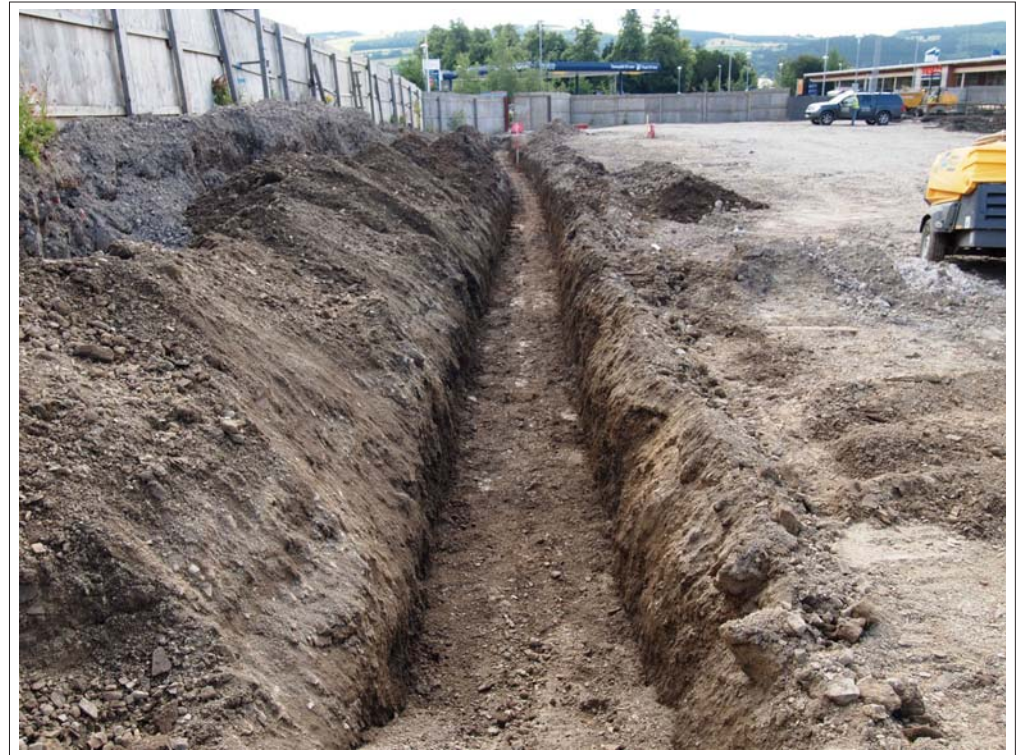
Plate 14 - Service trench, view south-east, 2m scale
