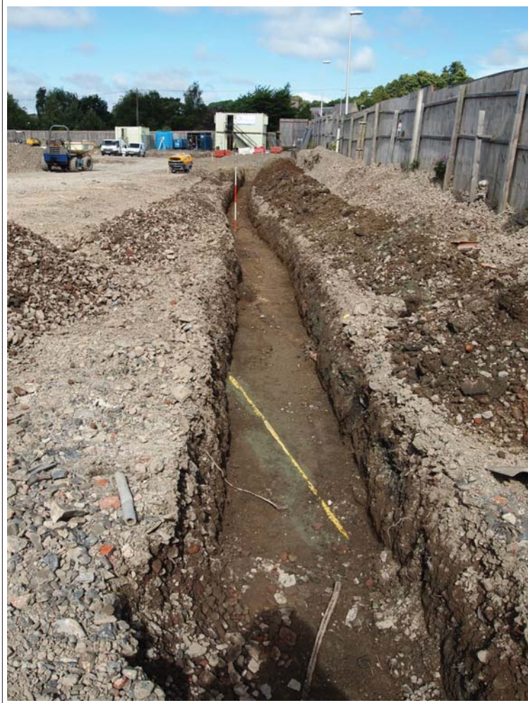
Plate 13. Service trench, view north-west, 2m scale
