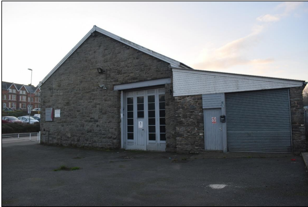
Fig. 3 North-east elevation of the goods shed showing through door for railway line and modern garage extension to the north-west (right of shot) Photo CPAT 4574-0002
