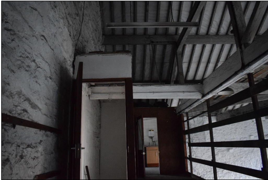
Fig. 7 Modern internal office structure within the goods shed, wooden lintel in visible in the stone wall of the shed adjacent to the staircase Photo CPAT 4574-0041
