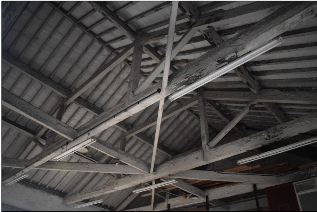
Fig. 5 Roof structure within goods shed Photo CPAT 4574-0019
