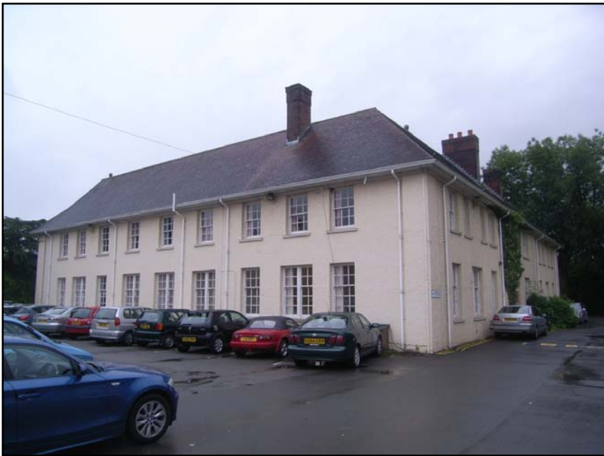
Plate 2 Rear/side elevations of F-Block (looking west)
