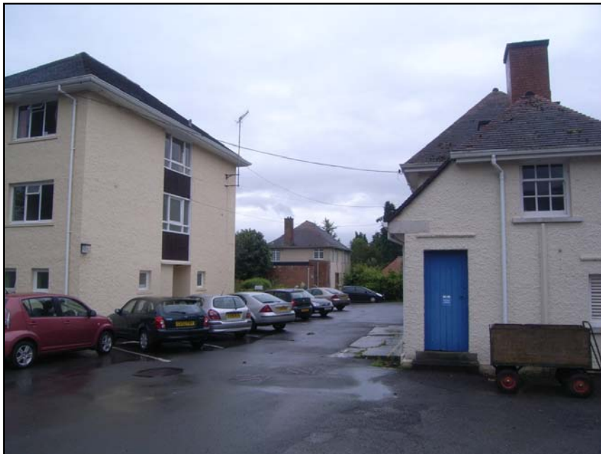
Plate 8 View south--east along access road - left foreground is B-Block and beyond is A-Block. Right foreground is north- east corner of J-Block
