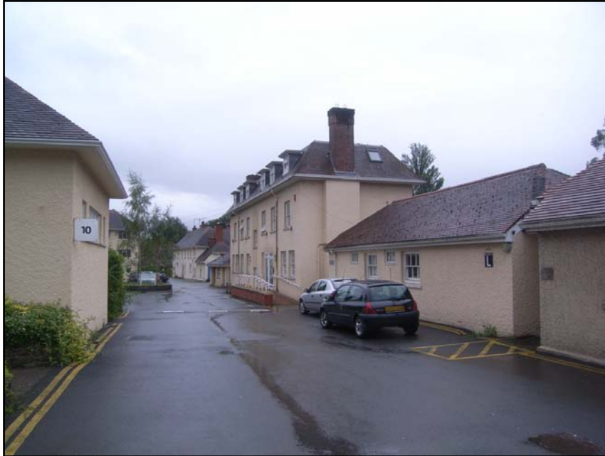
Plate 4 View south-east along access road - left fore- ground is E-Block and beyond is the south-west corner of B-Block. Right foreground is part of GL- Block, the rear elevation of H-Block, the north- east end of I-Block and J-Block
