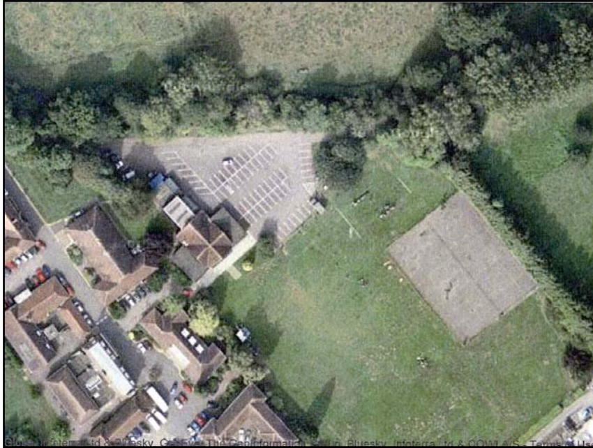
Plate 10 Site A - the proposed location for New Sports Hall (© Google Earth)
