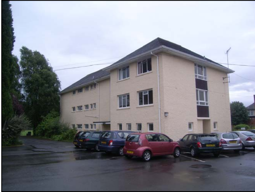
Plate 7 Front/side elevations of B-Block (looking east)
