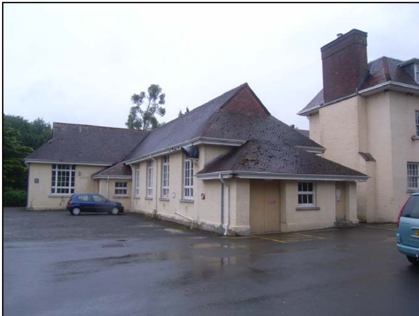
Plate 5 Rear elevation of I-Block (looking west)
