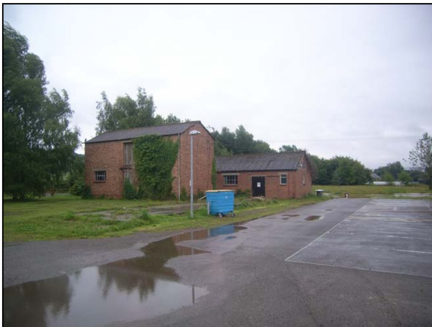
Plate 12 Site B - proposed loca- tion for Phase 1 'LRC, Café, Teaching and Admin' block, currently occupied by two redund- ant brick buildings (looking east)
