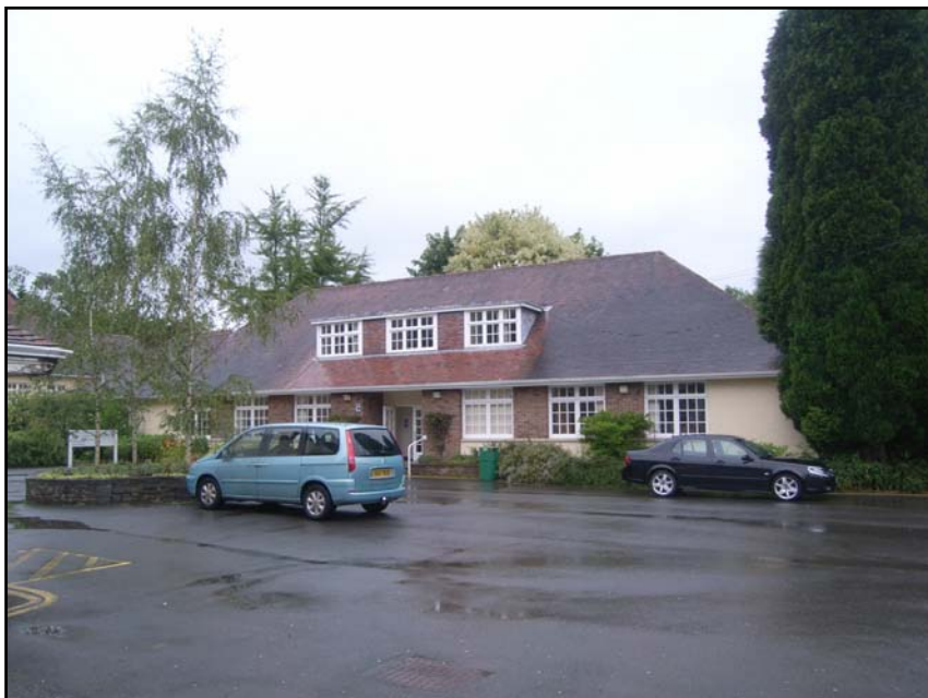
Plate 6 Front elevation of C- Block (looking north-east)
