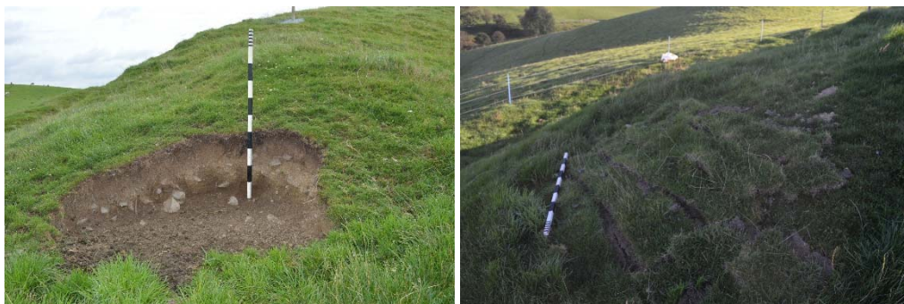
Fig. 10 and 11. Sheep scrape on north-west extent of monument before and after repair work. CPAT 4224-0046 and CPAT 4224-0115
