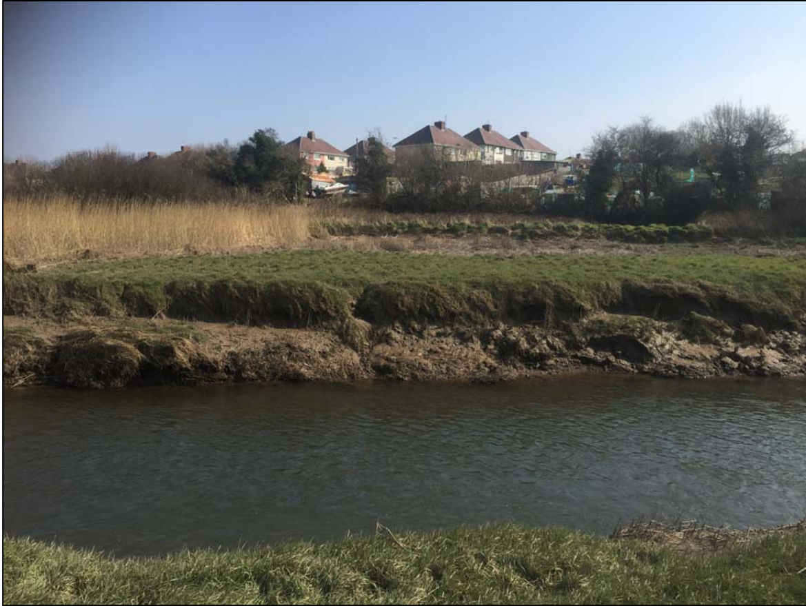
Plate 2: Looking across the Gwendraeth Fach to the earthwork bank, ID number 18, probably a flood defence on the other side.
