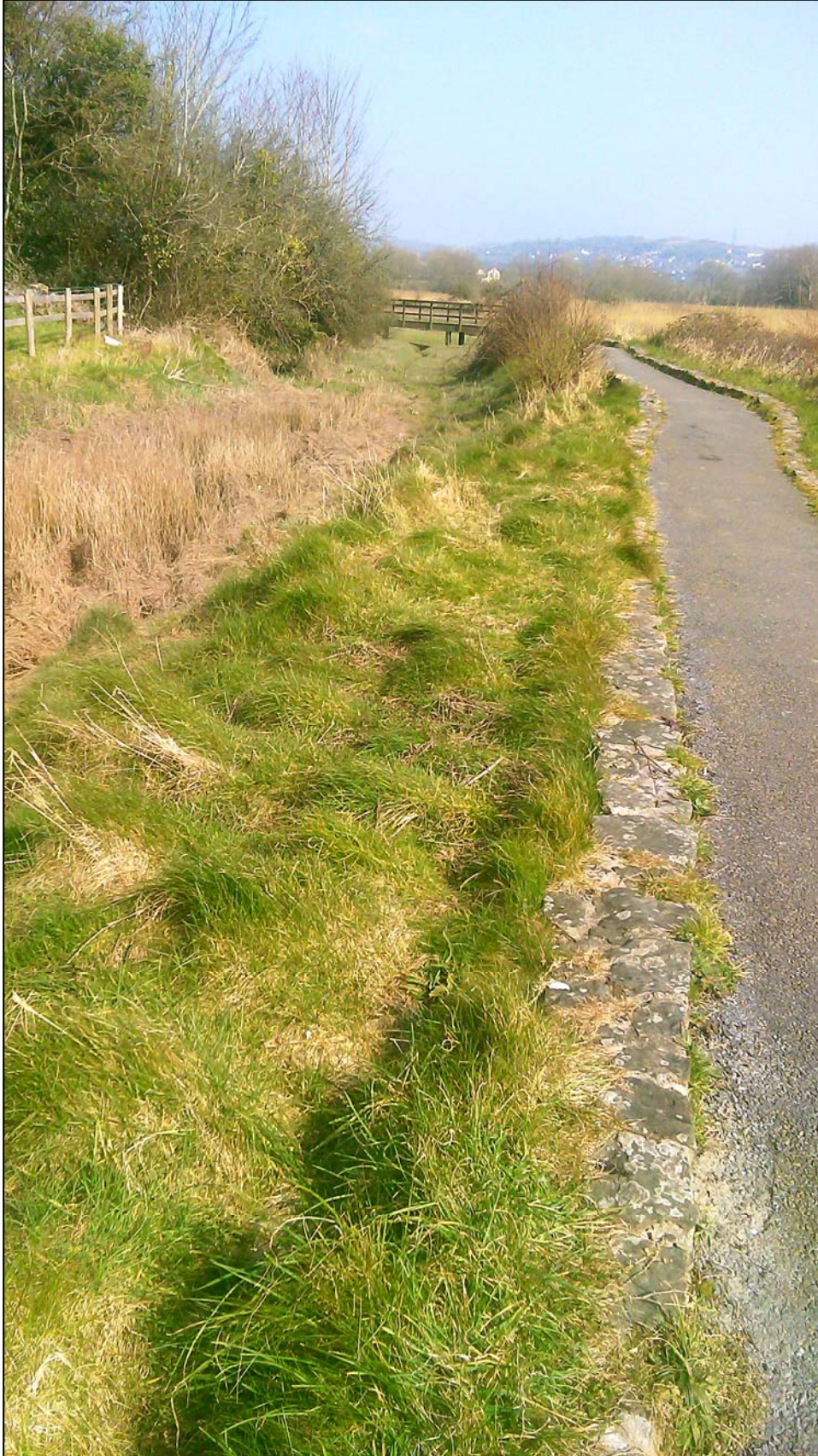
Plate 3: The leat, ID number 20, on the left hand side of the photograph with the more recent path that runs along its southern side, looking east.
