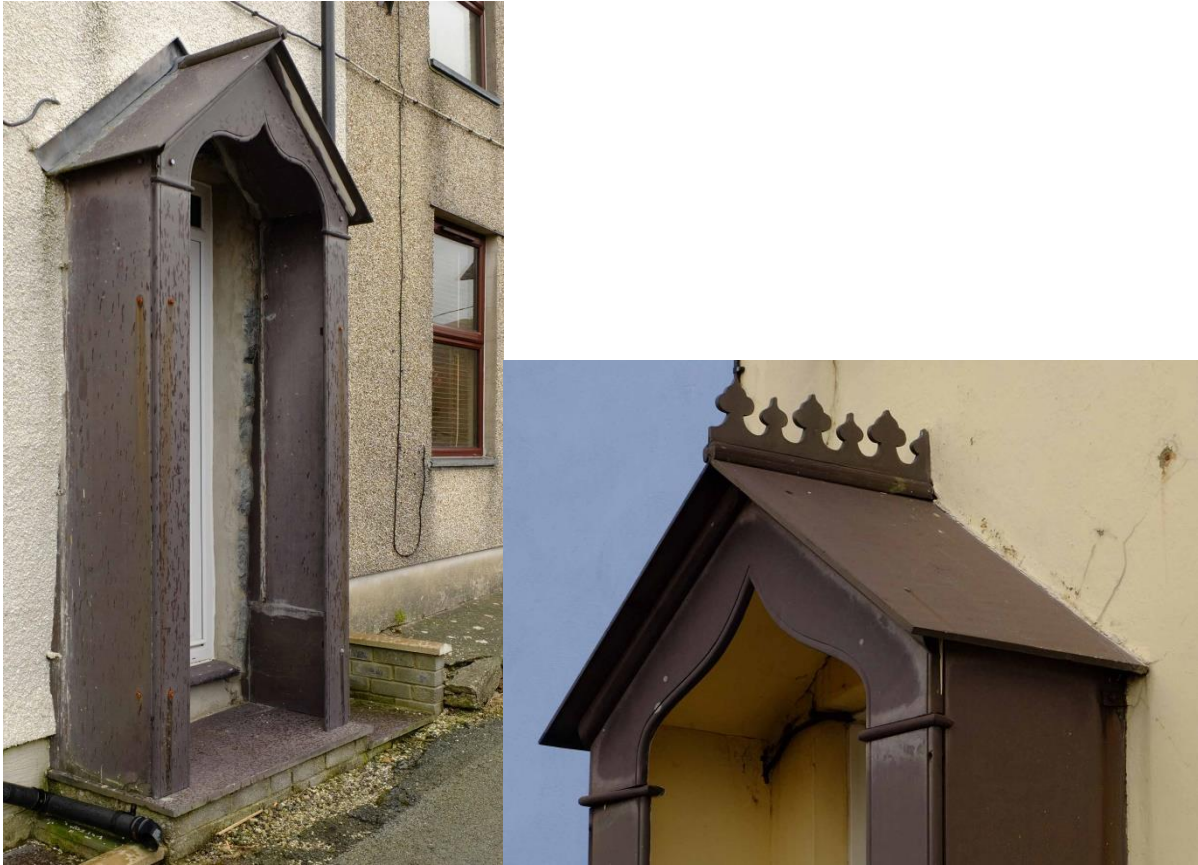
Fig 26 Slate porch details.
