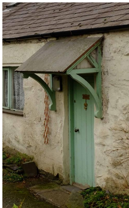
Fig 25 Slate-slab roof on a bracketed porch canopy.
