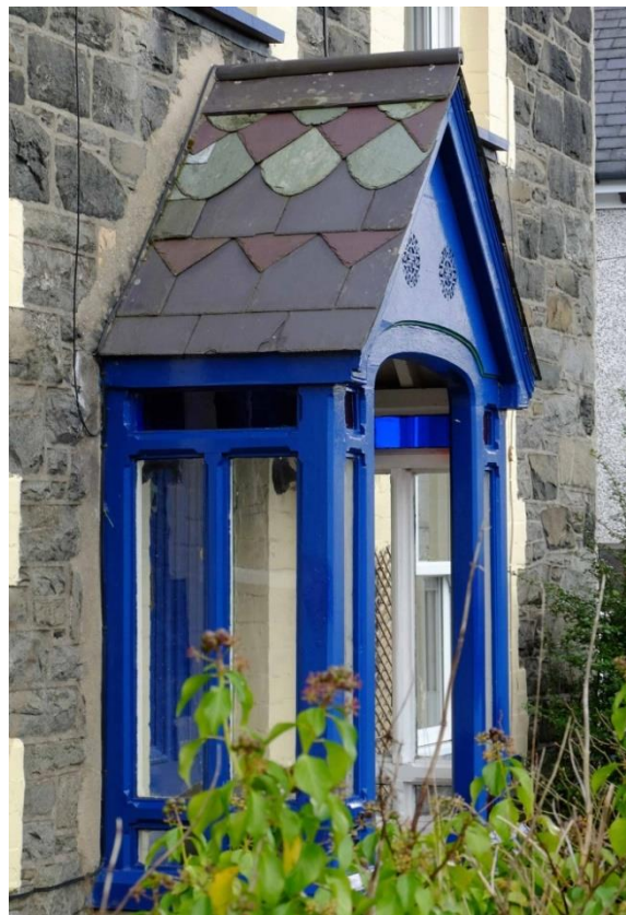
Fig 23 Shaped slates are uncommon, but are used here for picturesque effect on a wooden porch.
