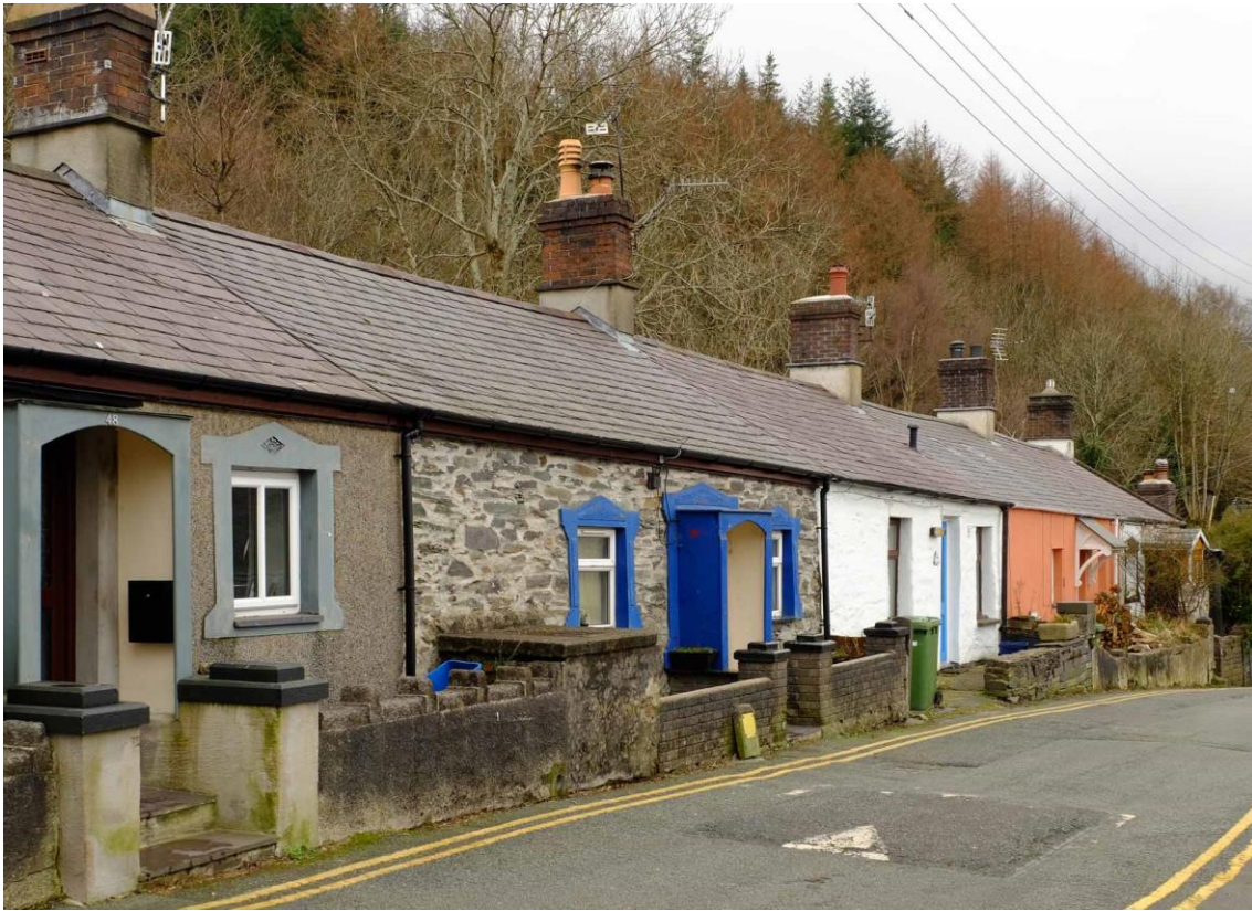
Fig 11 Single-storey cottages, Braichmelyn. These represent the earliest type of industrial housing. Garden walls and porches are a later addition.
