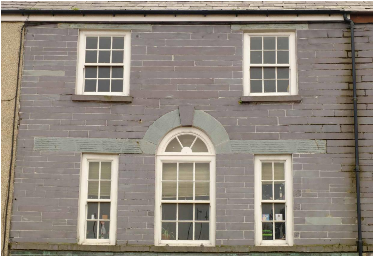
Fig 20 Number 2 Ogwen Terrace, originally a bank, distinguished by the Palladian arrangement of windows in the middle storey, under sandstone lintels and arch.
