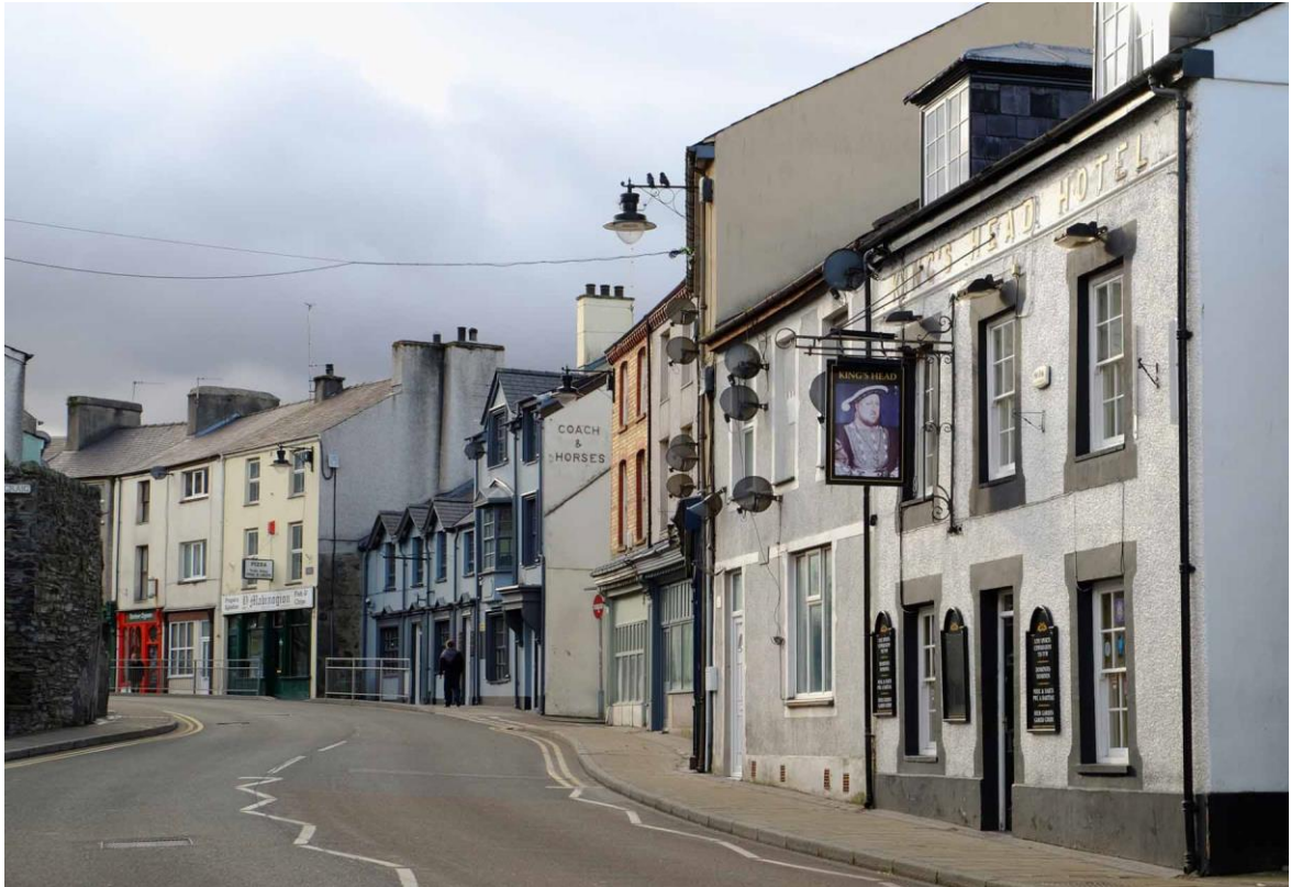
Fig 19 High Street, a mix of two-storey and three-storey commercial buildings
