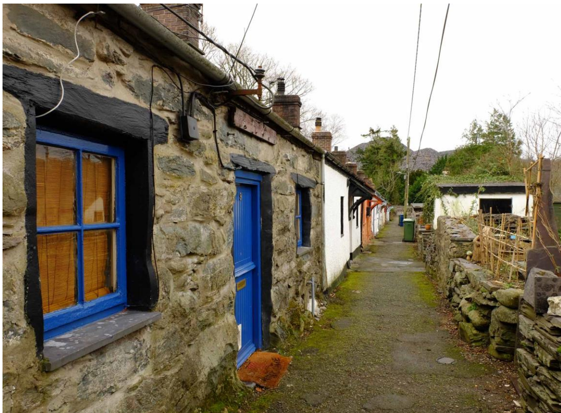
Fig 12 Caerberllan, built by 1840, with communal access path and gardens at the front instead of the rear. These gardens originally had stone-built coal bunkers.
