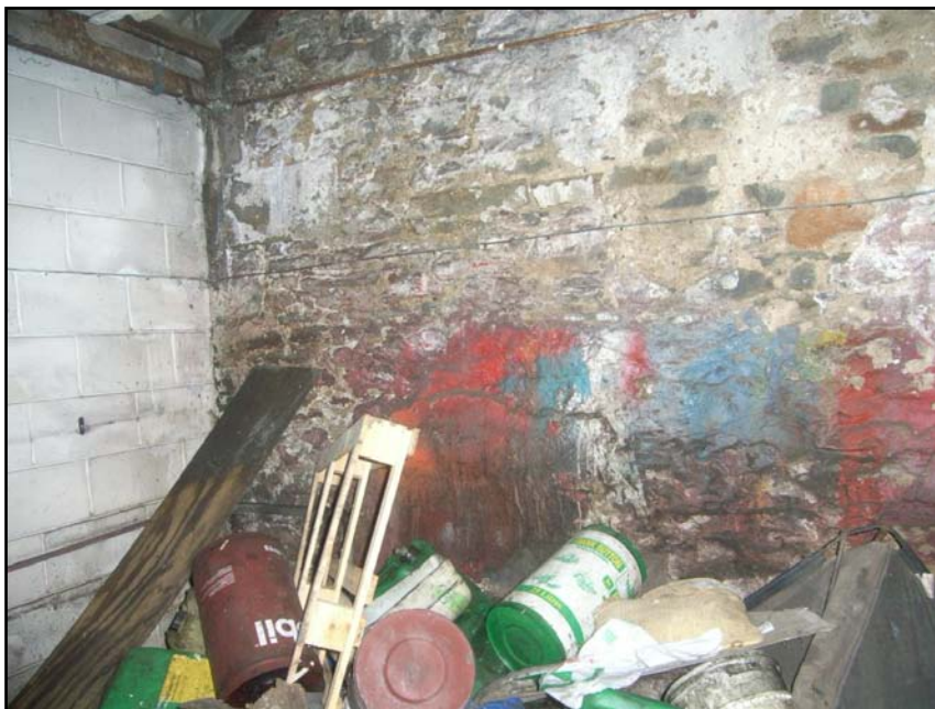
Plate 8 Inside of north wall: west end with blocked alcove
