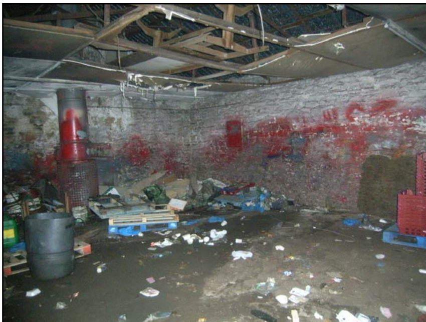
Plate 6 General view of interior, looking north-east
