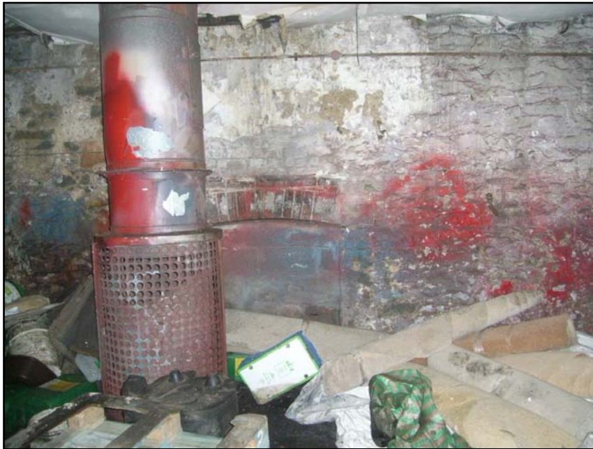
Plate 7 Inside of north wall: centre, showing blocked fireplace, also gas burner
