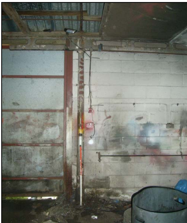
Plate 9 Iron column and portions of perforated lintel
