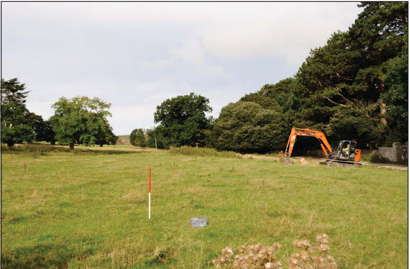
Plate 2: Wide angle view showing evaluation area pre-ex with garden boundary wall to the north; scale: 1x1m (archive reference: G2571_009).
