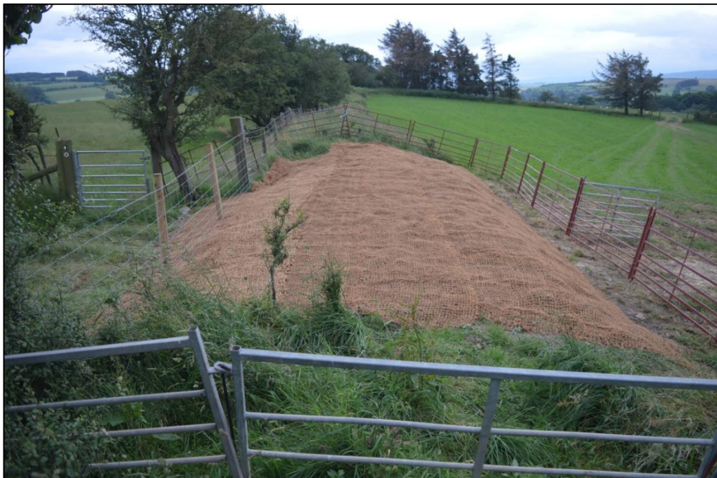
Fig. 9 The reinstated section of the Dyke following laying of the stabilising matting, viewed from the north. Photo CPAT 4663-039
