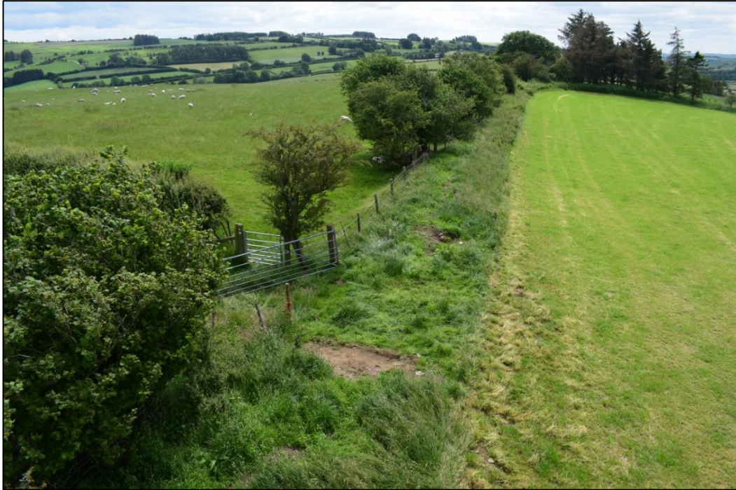
Fig. 3 Extent of damage to the Dyke viewed from the north. Photo CPAT 4663-004
