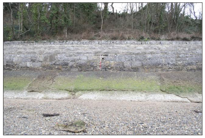
Drain Type 2: Circular pale orange ceramic pipe bonded into the wall construction with concrete between point E and point F. Diameter of pipe is 0.12m / 4 inches. Scale 1x1m.
