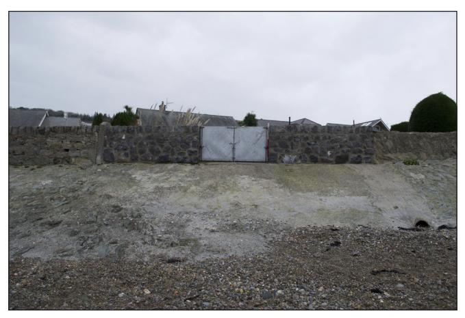
Drain Type 6: Circular pale grey concrete pipe partly subsumed located at the base of the wall slope to the immediately north of (point E) Flood Gate No.7. Diameter of pipe is 0.30m / 12 inches. Scale 1x1m.
