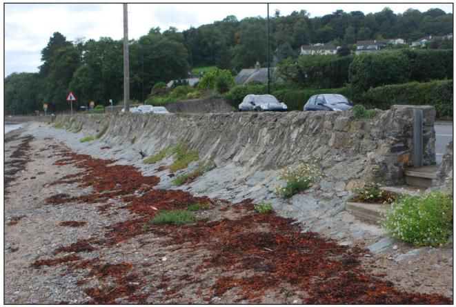
Plate 13: View of the concave rear face of the sea wall at point D (Flood Gate No.6). Photograph taken from the beach.
