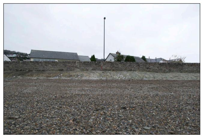
Plate 20: View of the concrete poured over the sloping sea wall between point E and point F. Photograph taken from the beach. Scale 1x1m.
