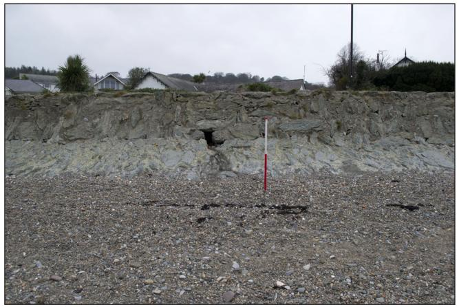
Drain Type 1: Narrow drain constructed as an integral part of the wall design between point C and point E. Individual dimensions vary from drain to drain. Scale 1x1m.
