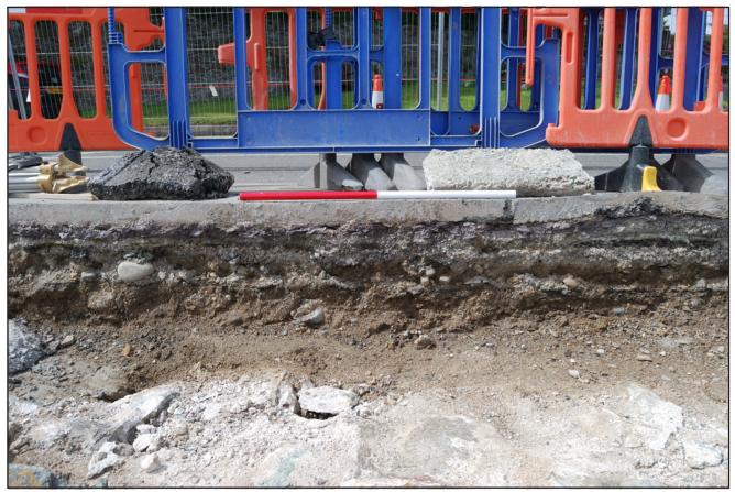
Plate 27: Cross section of the A545 road between point E and point F. Note the large beach rolled stone within the section to the left of the ranging pole. Photograph taken from the beach. Scale 1x1m.
