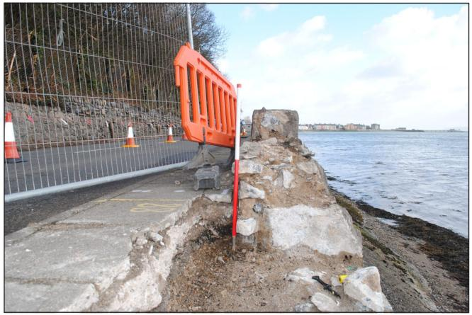
Plate 23: Representative cross section of the sea wall between point E and point F during its demolition. Scale 1x1m.
