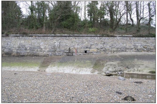
Plate 22: View of the join between two late phases of sea walling marked by the use of larger stone blocks between point E and point F. Photograph taken from the beach. Scale 1x1m.
