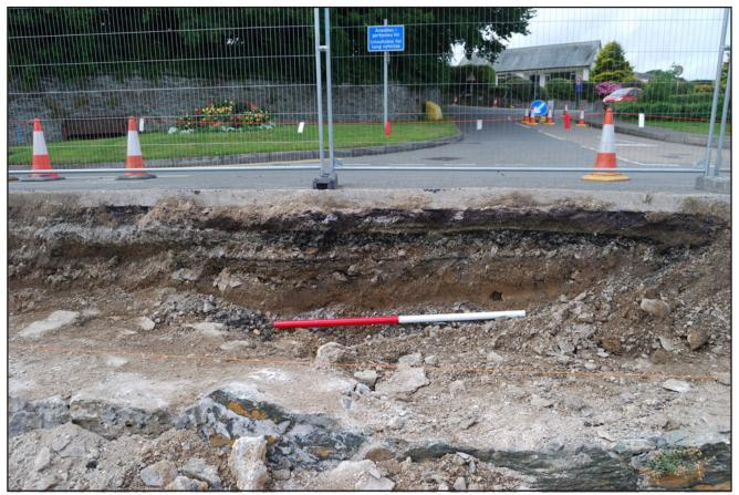
Plate 26: View of the deepest cross section of the A545 road between point E and point F. The clay layer immediately above the ranging pole may represent the base of the 1828 turnpike road. Photograph taken from the beach. Scale 1x1m.
