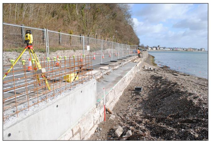
Plate 24: Representative view of the construction details of the new sea wall constructed on top of the earlier sea wall between point E and point F. Photograph taken from the beach. Scale 1x1m.
