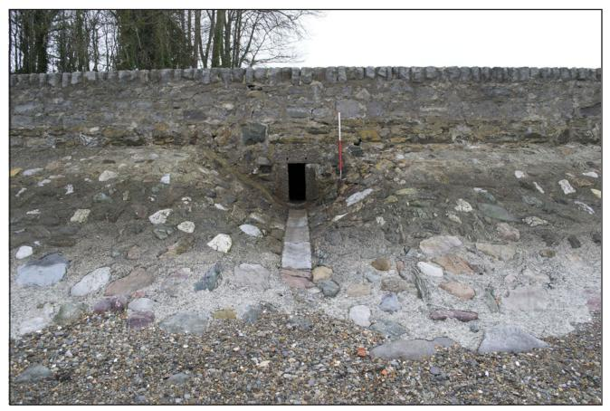
Drain Type 3: Narrow drain constructed as an integral part of the wall design between point E and point F. Taller and more elaborately constructed than a Type 1 drain and also chronologically later than a Type 1. Slate lined base to channel leading from the drain visible on the south western of the two examples. Individual dimensions vary between both drains. Scale 1x1m.
