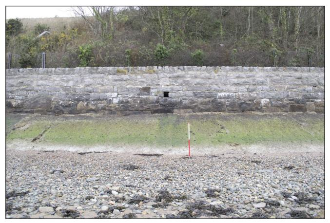
Drain Type 4: Square drain constructed as an integral part of the wall design between point E and point F. Individual dimensions vary from drain to drain. Scale 1x1m.
