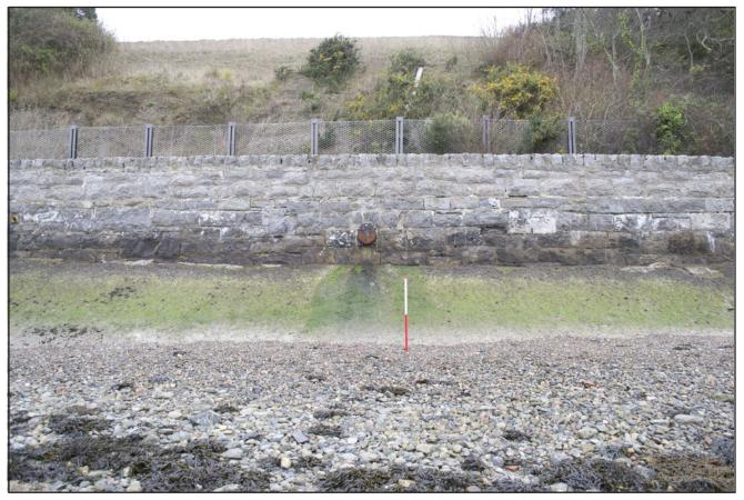
Drain Type 5: Cast Iron pipe with a top hinged cover. Writing on the hinged cover is 'HBH 300 DIA'. Located between point E and point F. Scale 1x1m.
