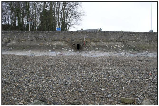
Plate 21: View of the early phase of sea walling around the southern of the two Type 3 drains and extending under the later phase of sea walling. Photograph taken from the beach. Scale 1x1m.
