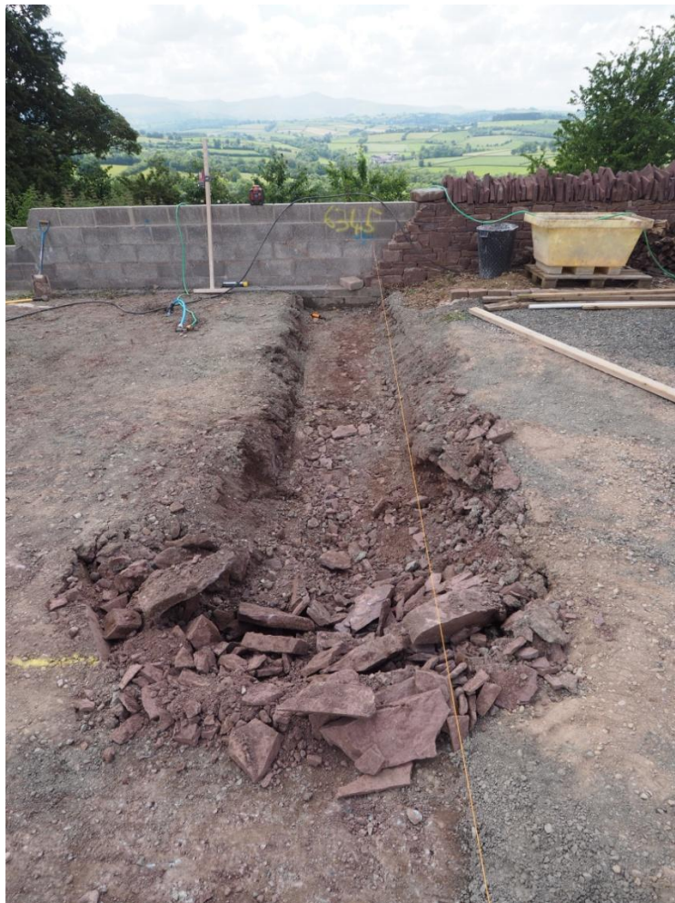
Figure 7: Trench A on completion of excavation
