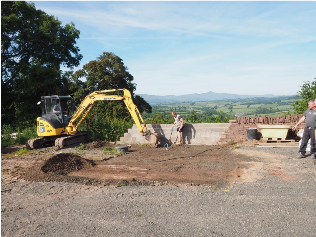
Figure 4: Stripping of scalplings layer
