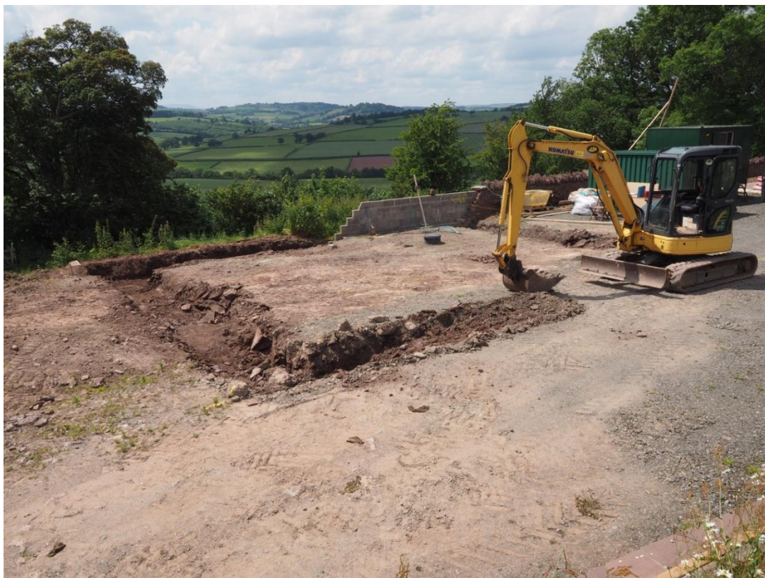
Figure 5: Completion of excavation of the foundation trenches
