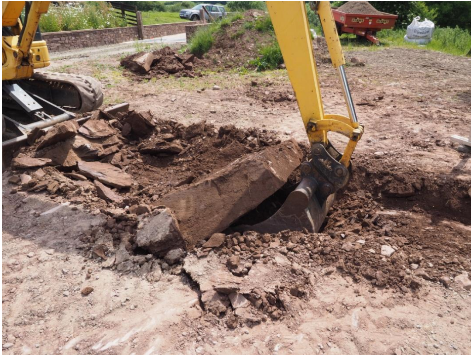
Figure 6: Trench C during excavation showing the nature of the bedrock
