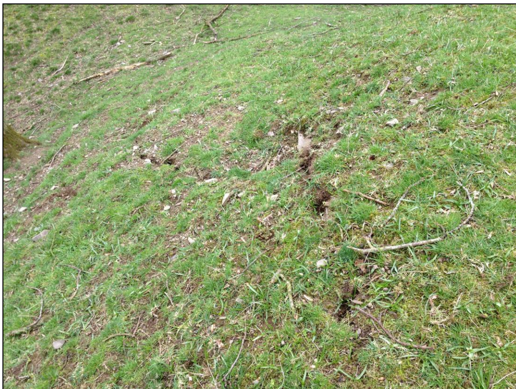
Fig. 22 Tomen Madoc, viewed from the south-west, showing surface cracking Photo CPAT 3808-0119
