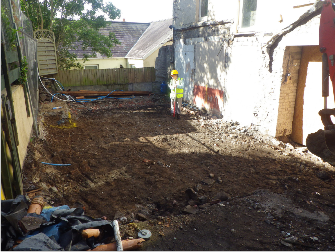
Plate 1: SRL2014_10, After removal of floors from previous extensions, looking southwest.
