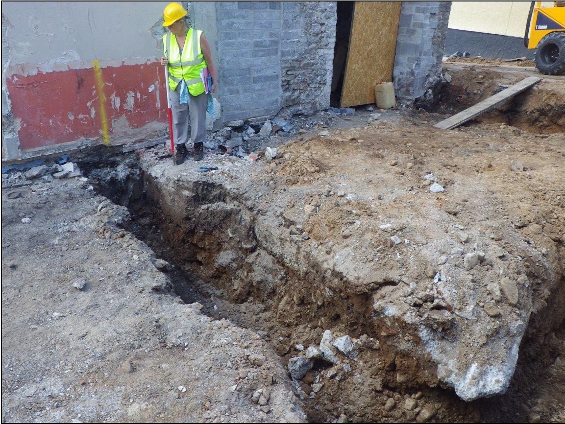
Plate 13: SRL2014_113, general view across foundation trenches, looking west.
