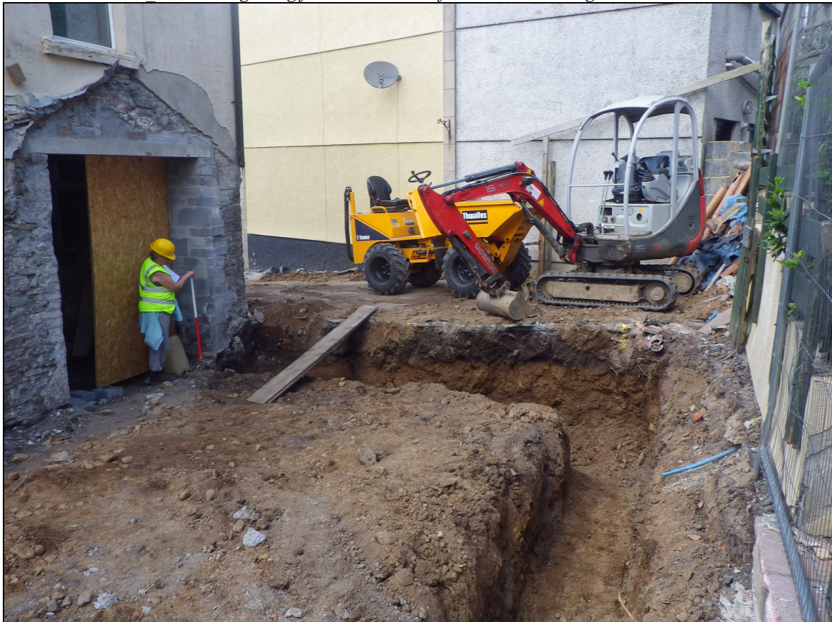
Plate 12: SRL2014_112, general view across foundation trenches, looking northwest.
