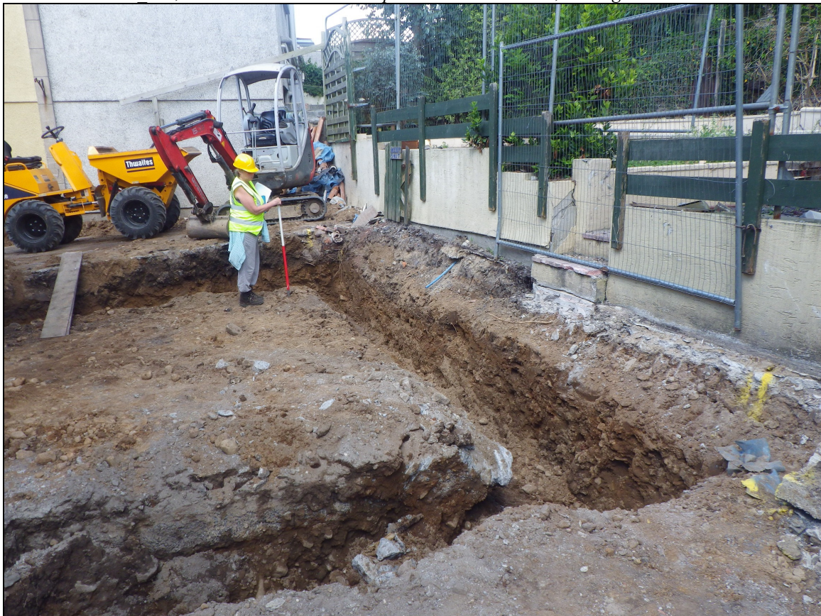
Plate 10: SRL2014_110, general view across foundation trenches, looking north northeast.
