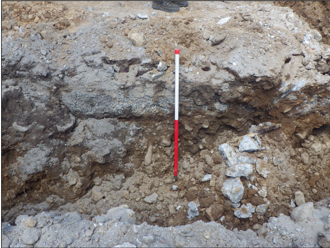
Plate 9: SRL2014_109, Foundation trench at mid point between A and B, looking north
