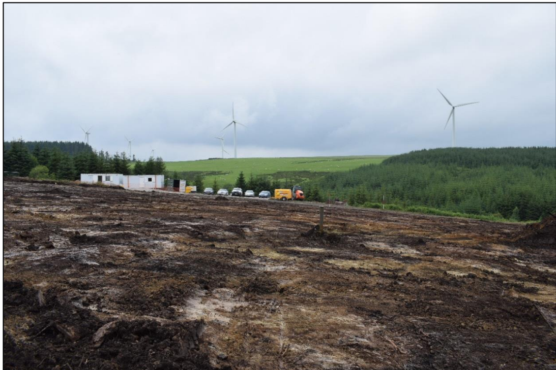
Fig. 3: The soil stripped area at the Clocaenog Substation, from the east. Photo CPAT 4362-0003.
