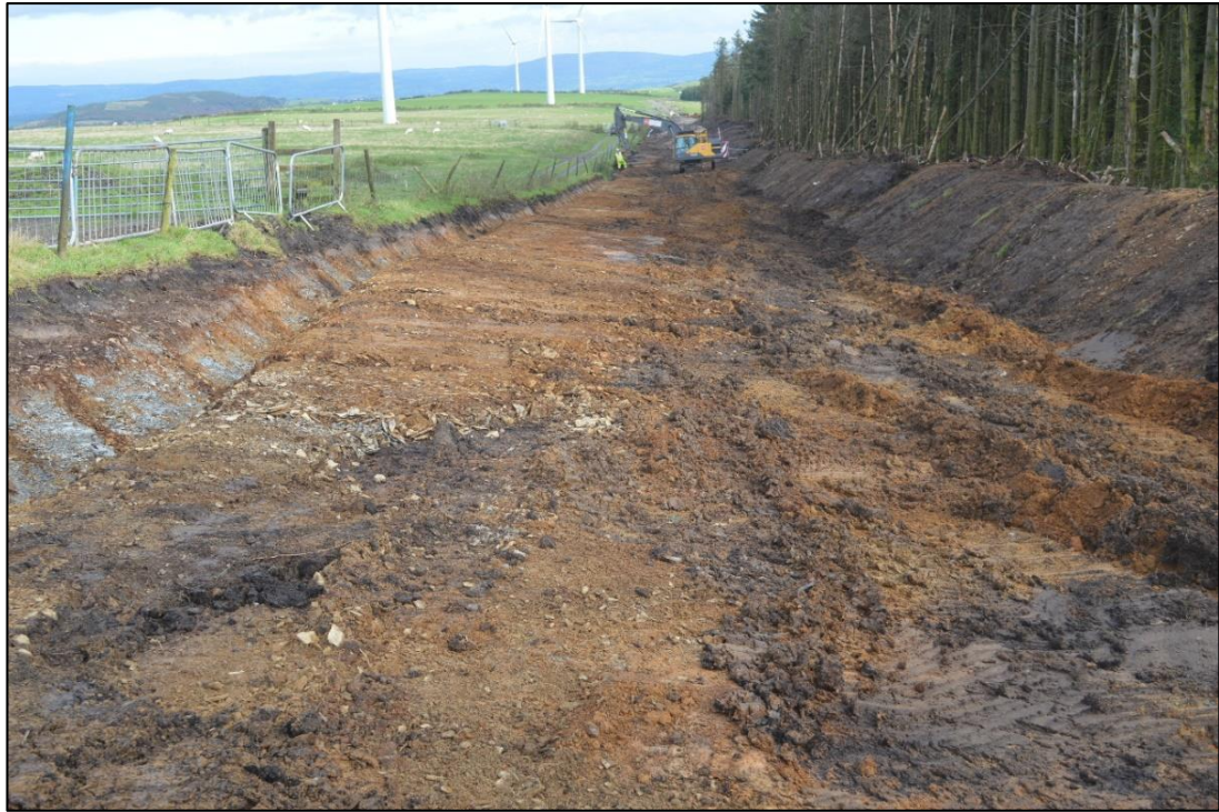
Fig 5: Phase 2 of cable trench, bordering pasture fields. Photo CPAT 4362-0011
