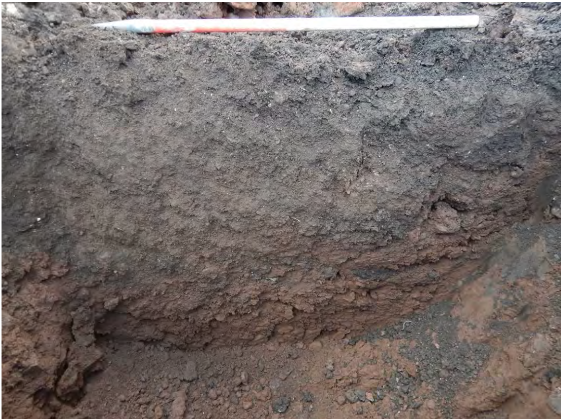
Photo 6: Northwest facing shot of the soakaway section. The depth prohibited cleaning, but topsoil (001) overlies deposit (002). 1m scale.
