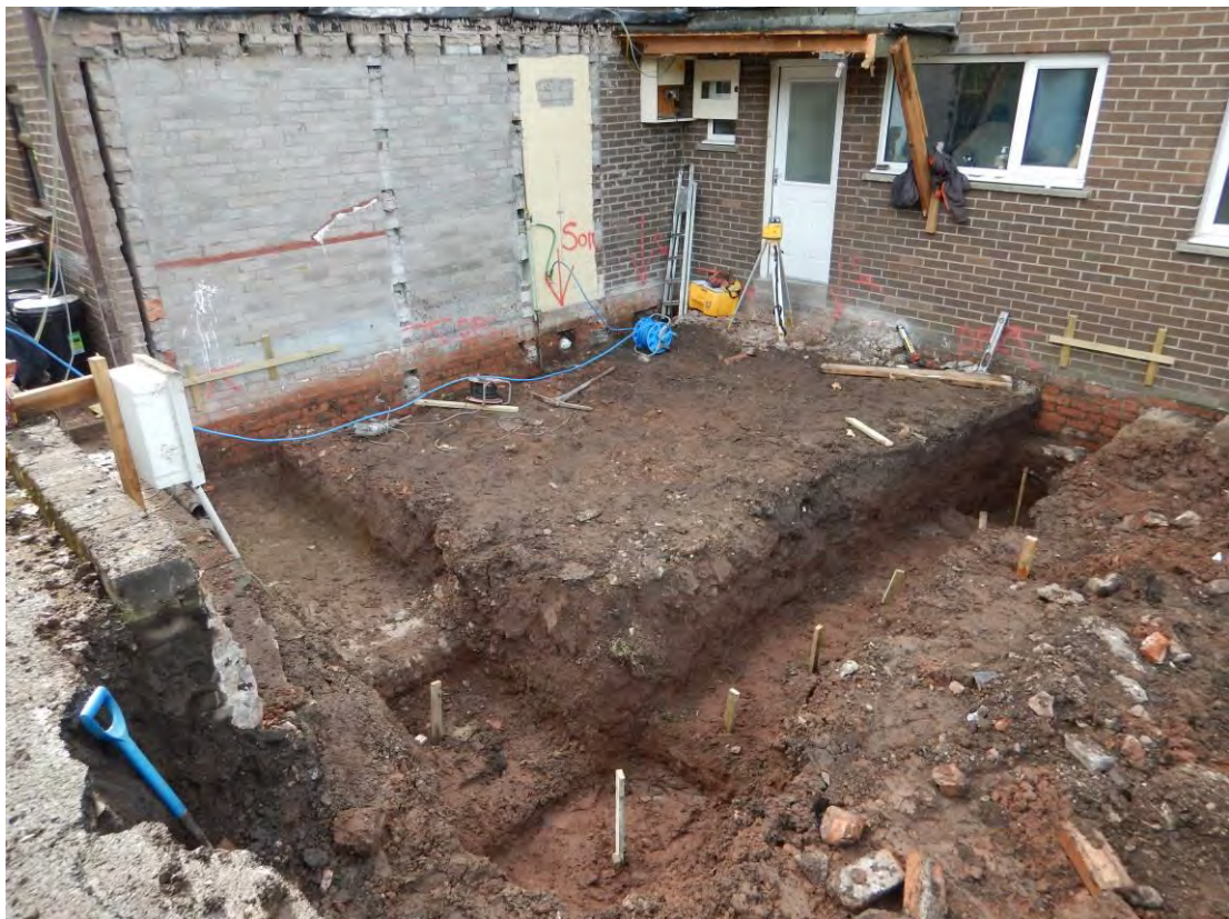
Photo 2: View southwest of the development site, showing excavated foundation trenches.
