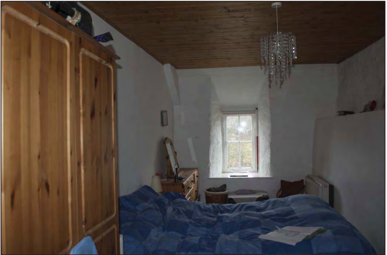
Plate 23: View of Bedroom 4 with a view of window W14, walled shelf and roof brace (photographic archive ref. G2520_046)
