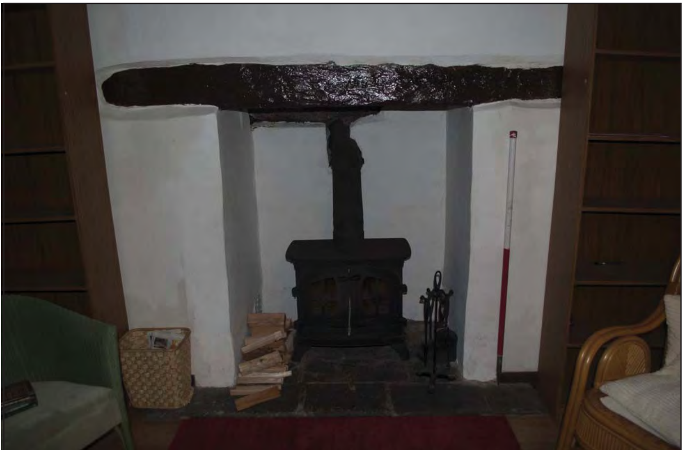
Plate 34: View of modernised fire range F01 within House 2, displaying original lintel (photographic archive ref. G2520_073)
