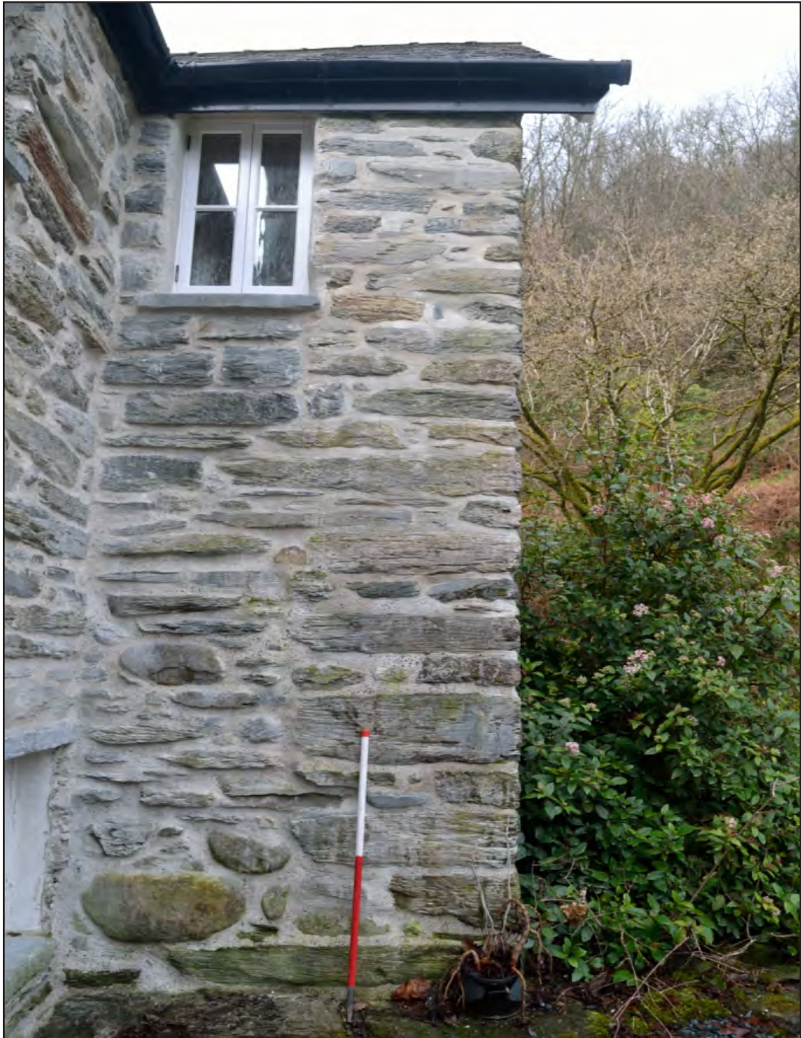
Plate 51: View of short SE facing elevation of House 1 showing small replacement casement window and blocked opening at ground floor level; Scale 1x1m (archive reference ; G2520_1108)
