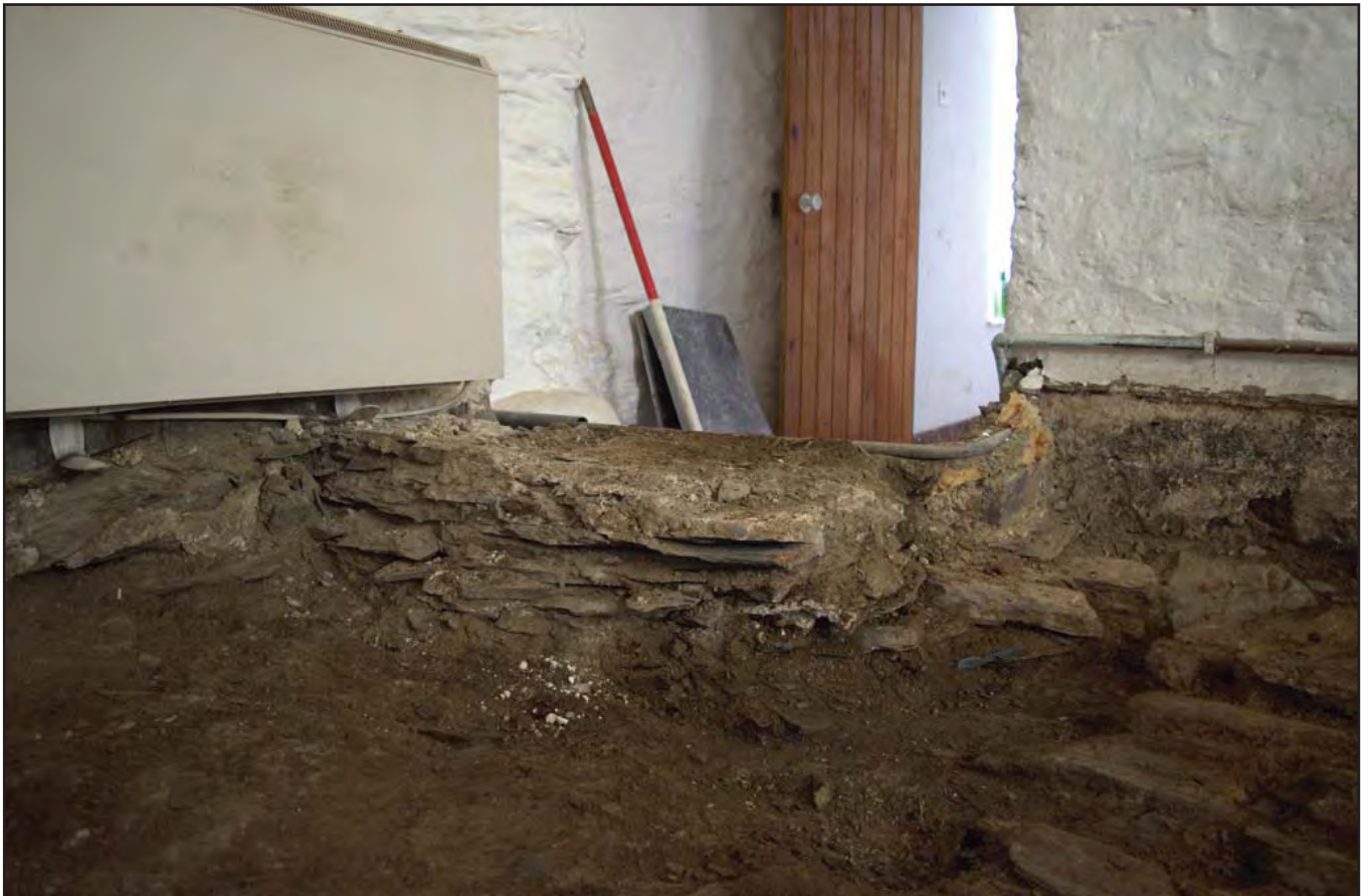
Plate 48: Step-up between living room and kitchen; scale: 2x1m (archive reference: G2520_1100).
