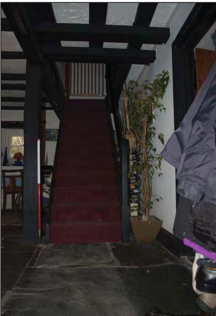
Plate 22: View of stair case with close up view of 18th/19th century slate floor against 20th century slate floor tiles (photographic archive ref. G2520_042)
