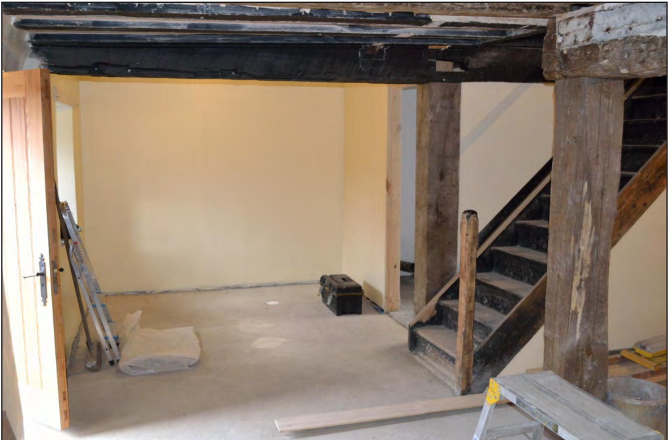
Plate 59: General view of Dining Room from Lounge 1 (House 1) showing the areas of panelling stripped out (archive reference: G2520_1123).
