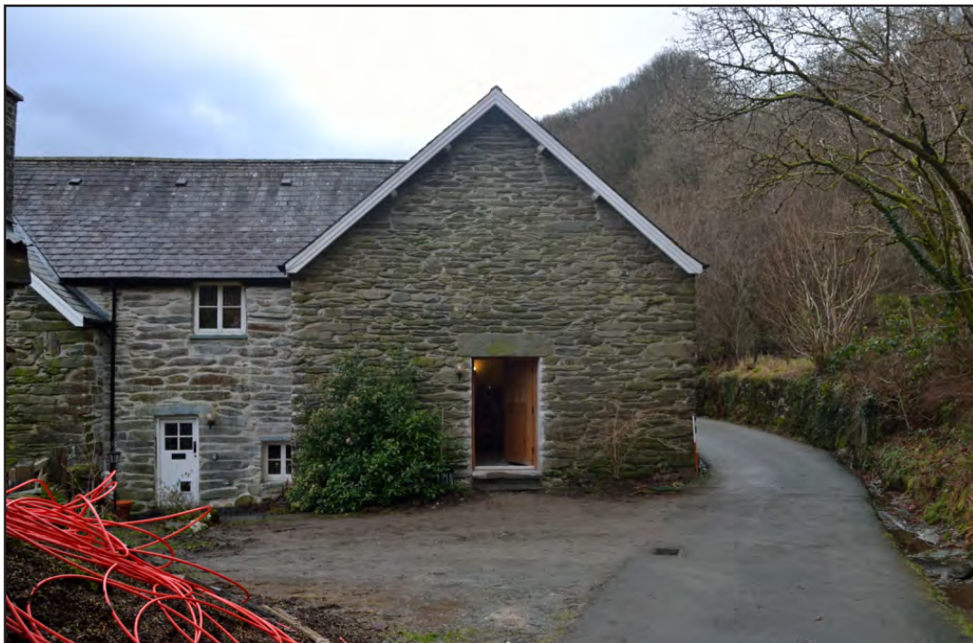
Plate 53: General view of north-east facing elevation of house 1 showing D04 open, with replacement timber panelled door; scale: 1x1m (archive reference: G2520_1117).
