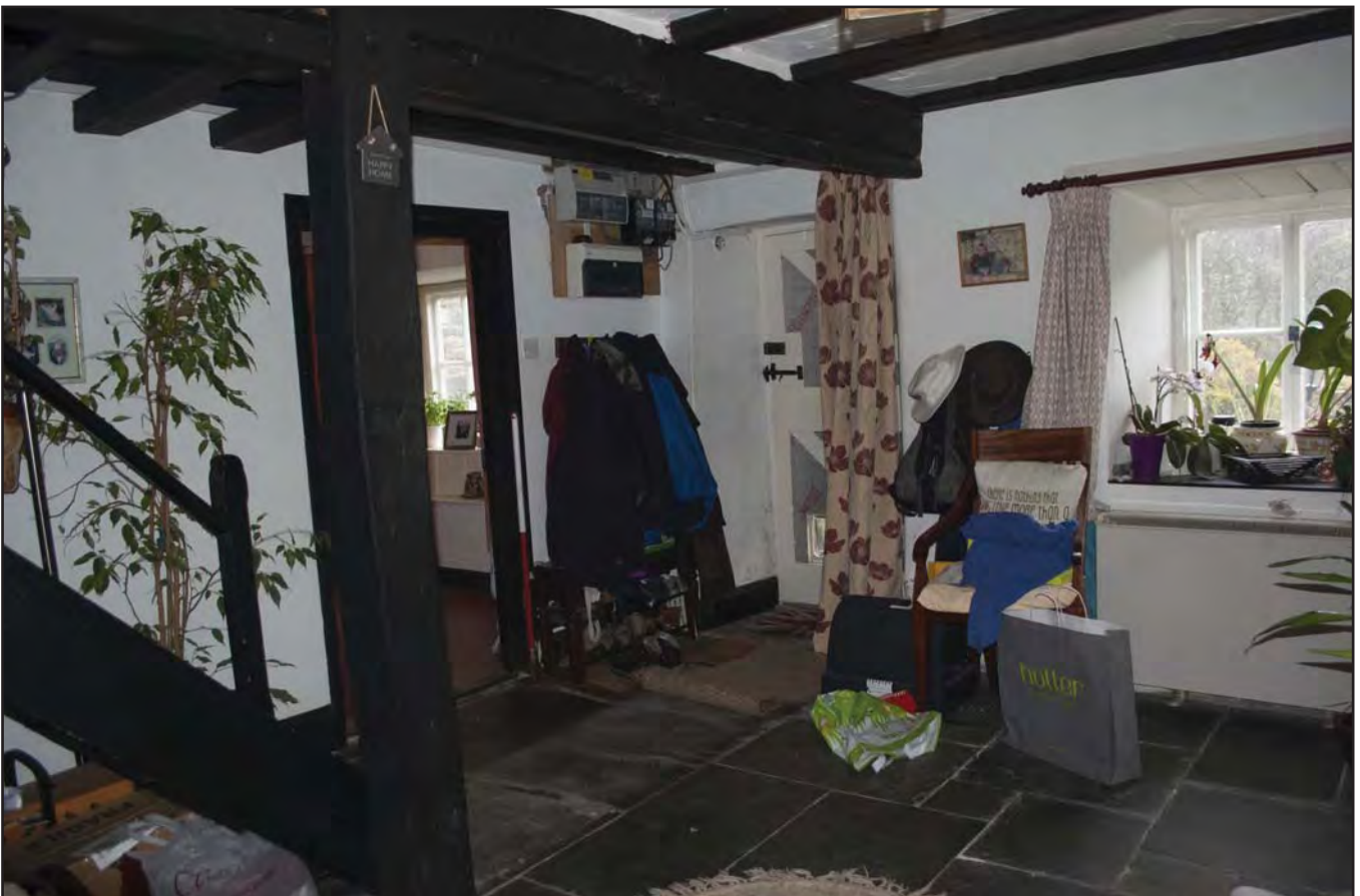
Plate 20: View of dining room with view of central beam running on west-east axis, alongside with view of two distinct phases of slate floor surfaces (photographic archive ref G2520_039)
