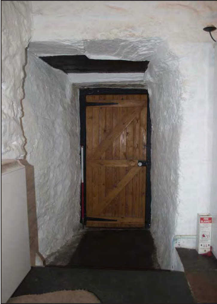
Plate 17: Passage entrance into the late 16th century house from Kitchen 1 into Lounge 1 (photographic archive ref. G2520_031)
