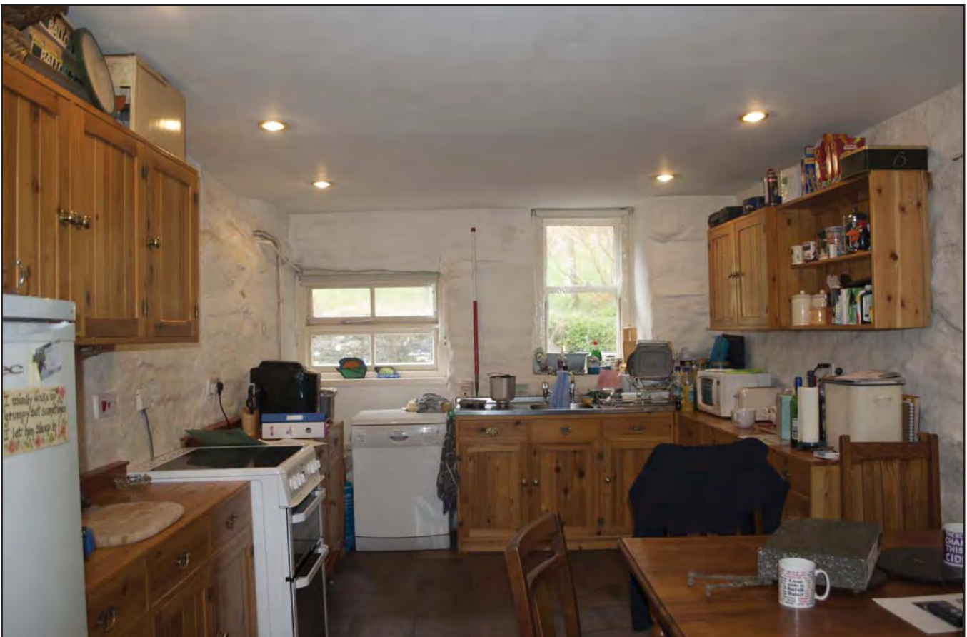
Plate 16: View of Kitchen 1 in House 1, showing evidence of later first floor expansion along east facing wall and former stairway window on the north facing wall (left). The return of doorway DB01 is visible alongside view of the 19th century window insertion of W01 (photographic archive ref. G2520_027)
