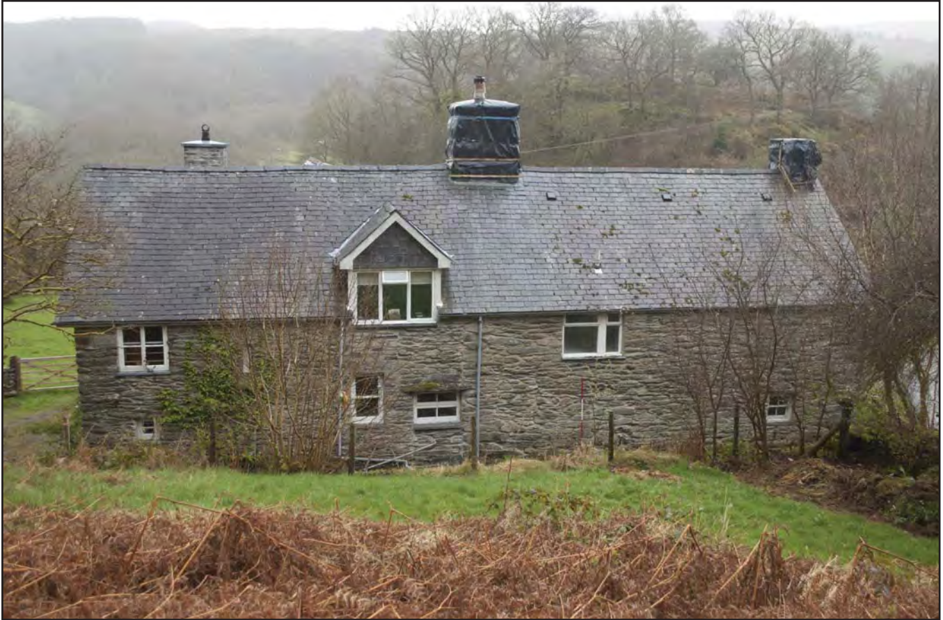
Plate 07: View of western elevation taken from raised ground at rear of Bryn Moel with view of chimneys and blocked window WB03 which may have provided light into the former 16th century stairwell (to the right of W02, formerly doorway DB02) (photographic archive ref. G2520_013)
