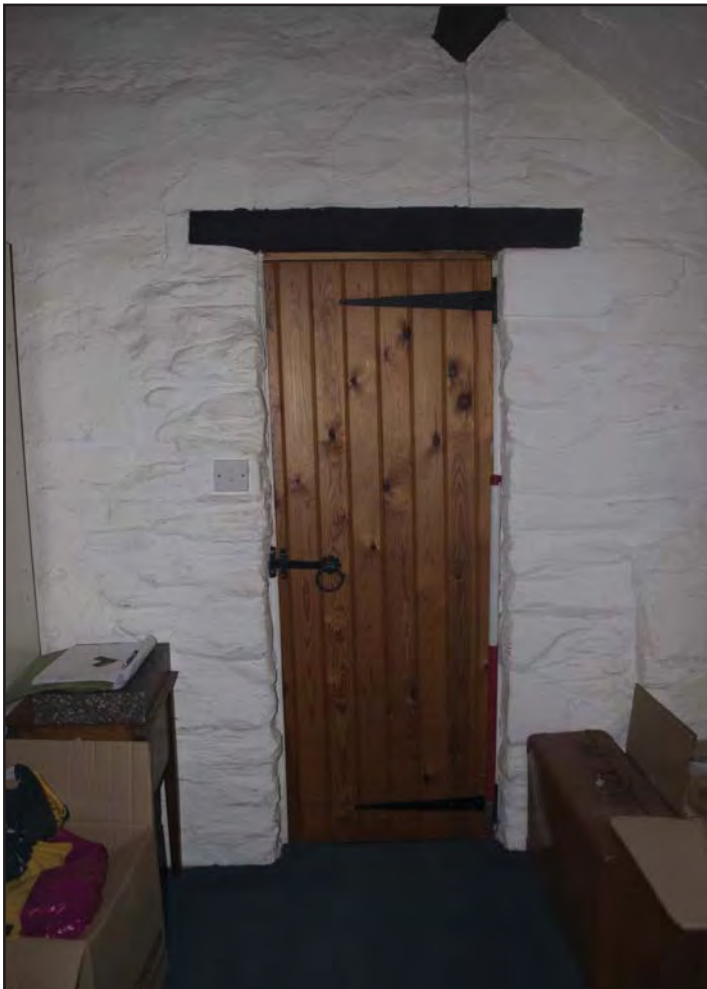
Plate 26: View of door D17 with lintel (photographic archive ref. G2520_061)
