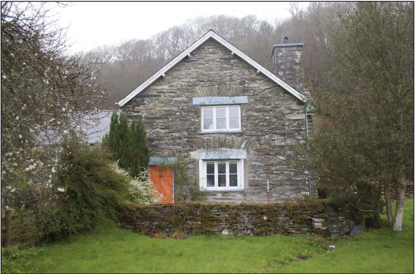
Plate 03: View of East gable end of House 2, with view of 17th century undressed segmented arched lintel above window W08 and later masoned flat arched lintel above W19 on the first floor (photographic archive ref. G2520_006)
