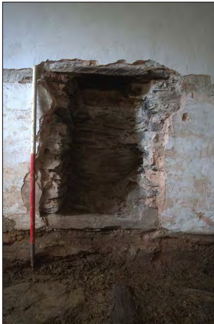
Plate 50: Fire place in the SW. corner; scale: 1x1m (archive reference: G2520_1040).
