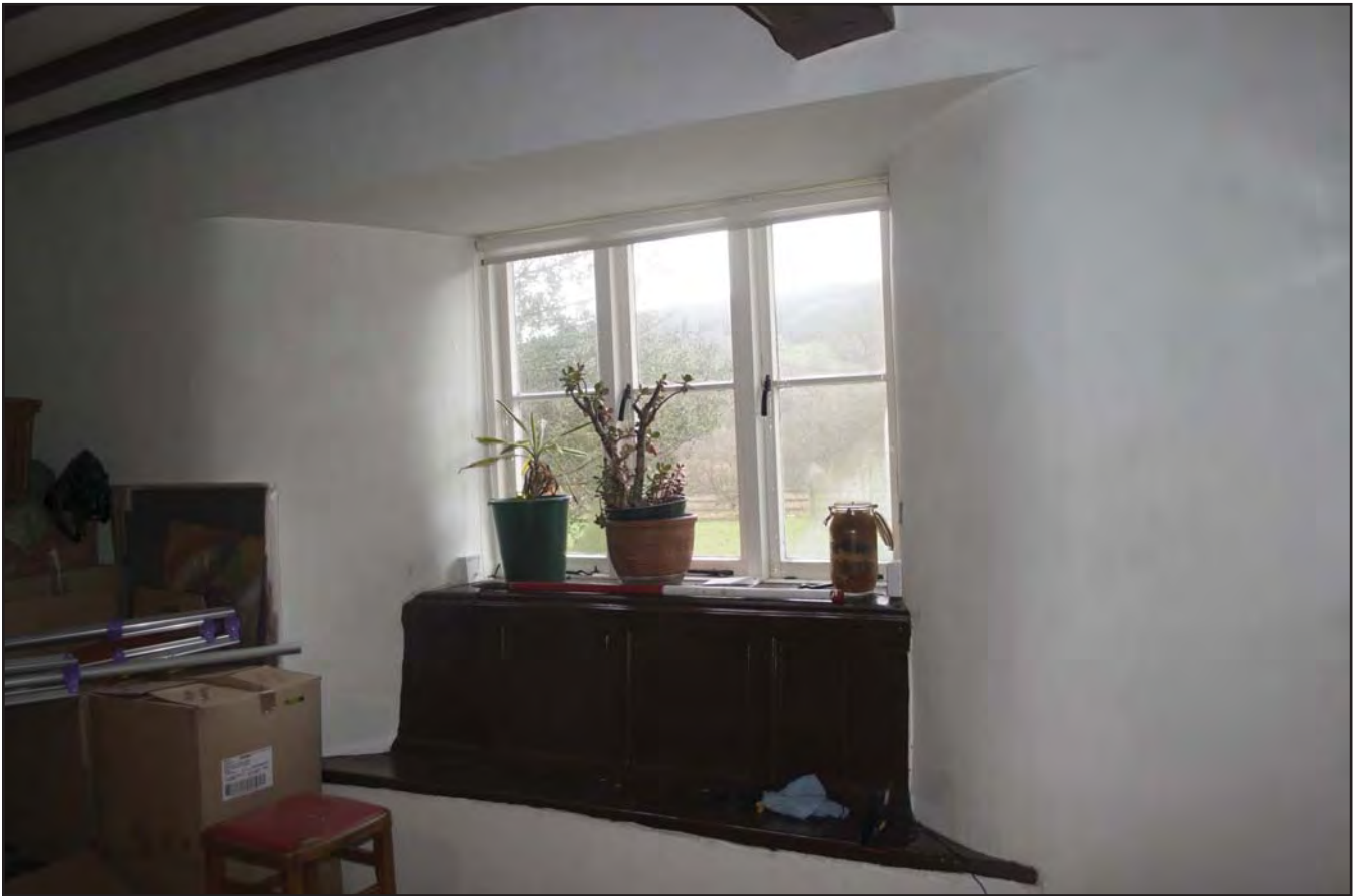
Plate 33: View of 17th century panelled window sill seat of window W08 (photographic archive ref. G2520_071)
