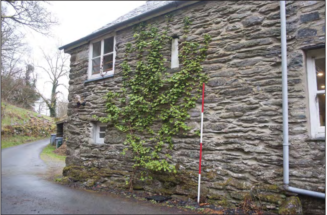
Plate 09: Oblique view of the north end of House 1's western elevation with view former barn ventilation window (WB04) in the 18th century northern extension (photographic archive reference G2520_016)
