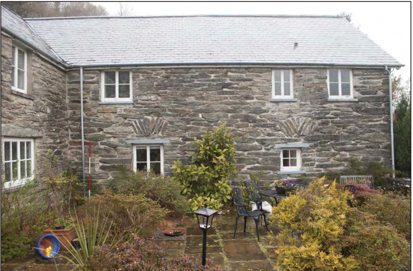
Plate 06: Close-up view of House 2 southern elevation displaying 17th century segmented arched lintels above former window W07 and cross passage doorway of W09, the faint line break of a later first floor extension is also visible (photographic archive ref. G2520_010)
