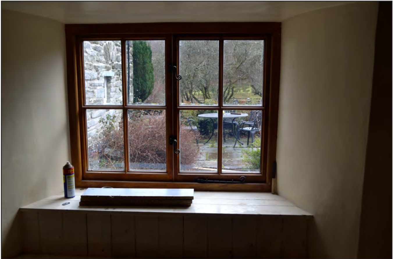
Plate 54: Internal view of W05, showing reveals and fitting (archive reference: G2520_1118)
