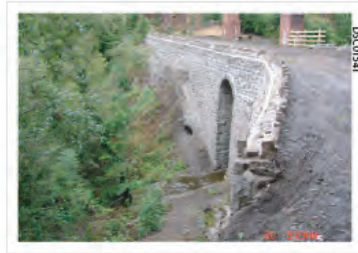
Plate 02: View over south revetment showing Hafod arch and storm arch
