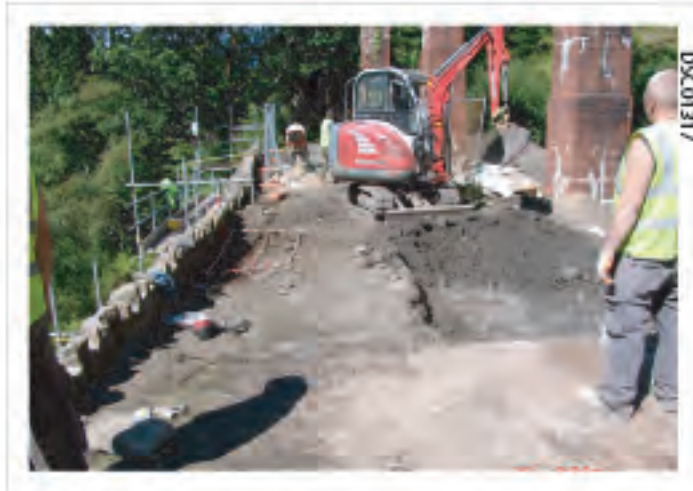
Plate 08: Excavation second cut trench 2 overview
