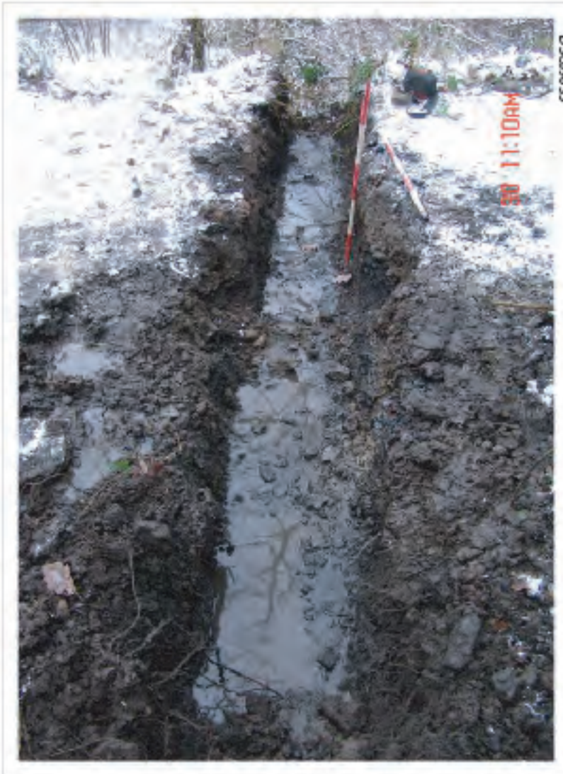
Plate 07: View across finished trench, water logging
