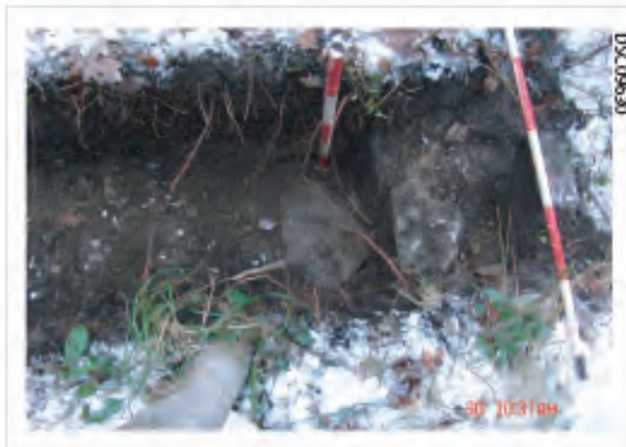
Plate 10: Buried section of south retaining wall in trench vertical 2
