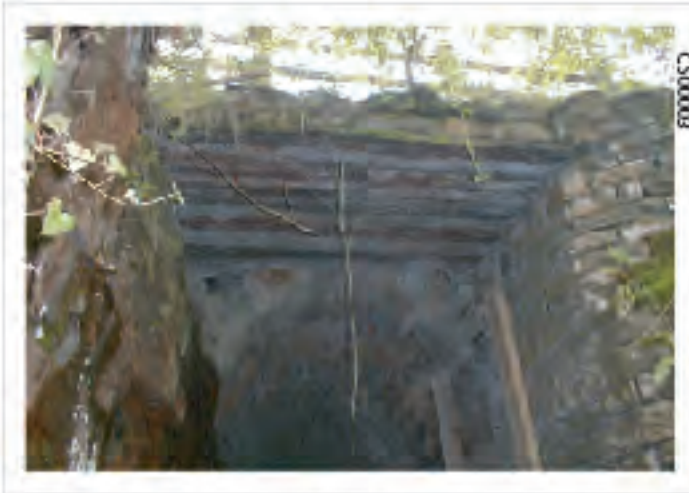
Plate 05: Earlier repair, Metal lintels.
