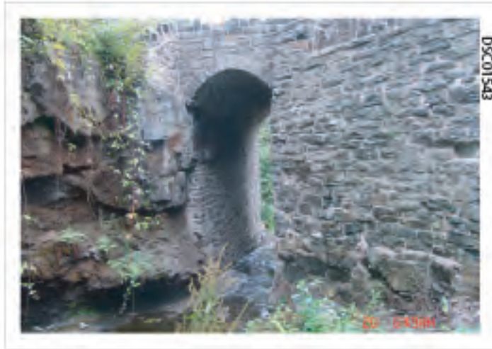
Plate 01: Northern side of Hafod arch showing butt to rock face and finished work
