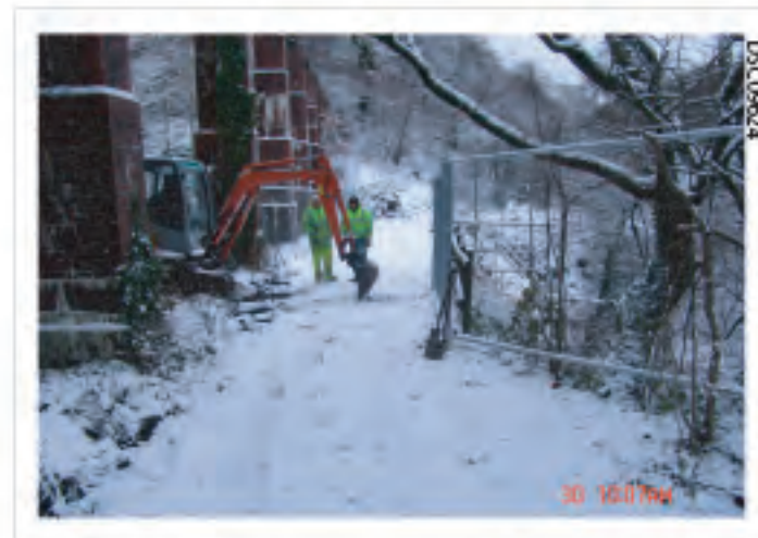
Plate 04: Beginning of excavation work, Trench 1
