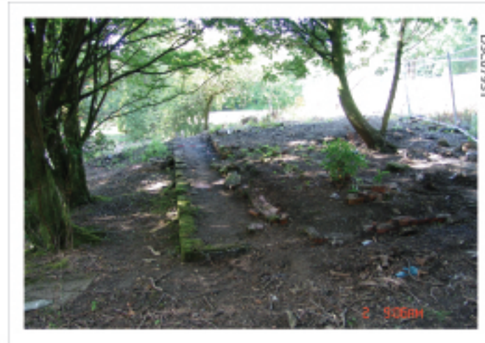
Plate 02: General view of structure before excavation
