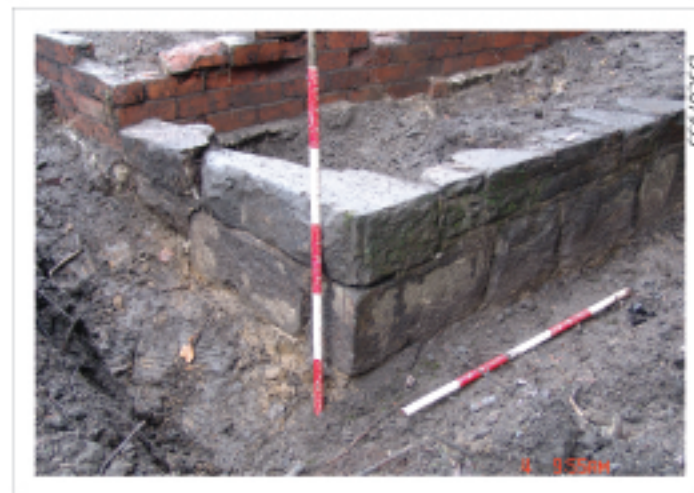
Plate 05: External wall at lower terrace SE corner showing dressed stone
