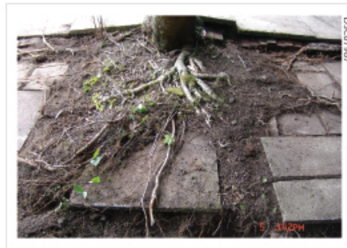
Plate 03: Mid and upper terraces.
