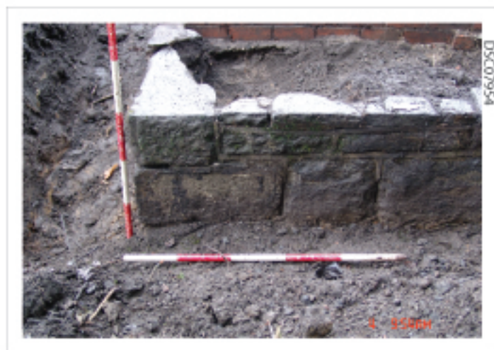
Plate 22: External wall at lower terrace SE corner showing dressed stone
