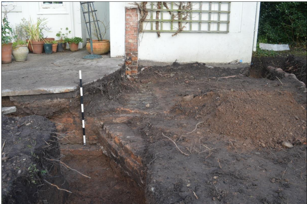
Fig. 5 Part of the 19 th -century culvert, with the scale against the brick wall of the cess pit. Photo CPAT 4579-0001
