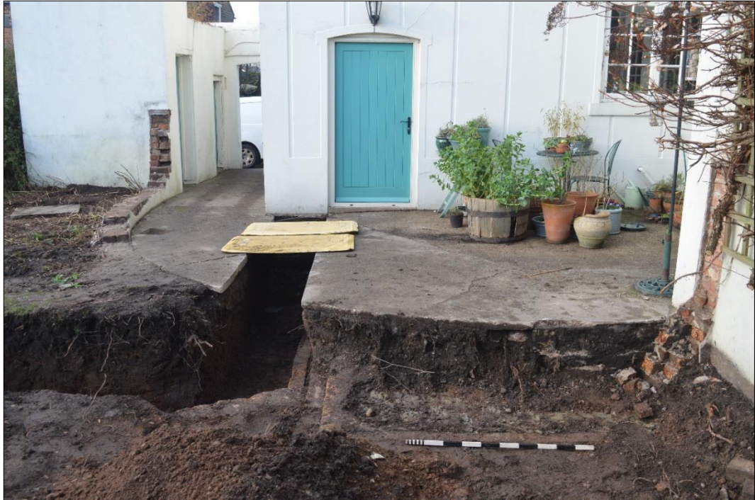
Fig. 6 Part of the brick-built cess pit, extending beneath the concrete patio. Photo CPAT 4579-0005
