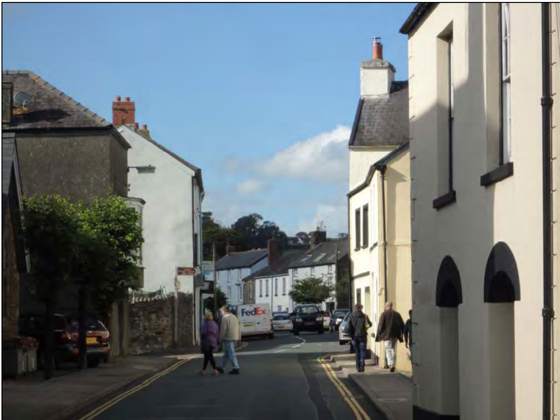
Plate 1: View northwards along King Street, Laugharne towards Glen View.
