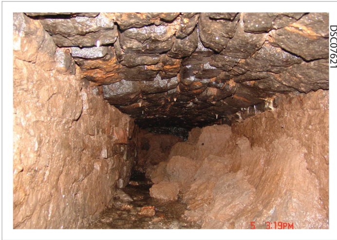
Plate 01: Silting within outfall
