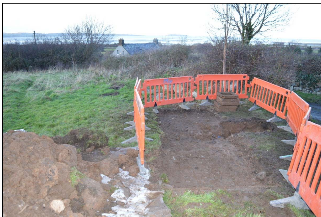
Fig. 02 Trial Pit 1, viewed from the south-east. Photo CPAT 3966-0006
