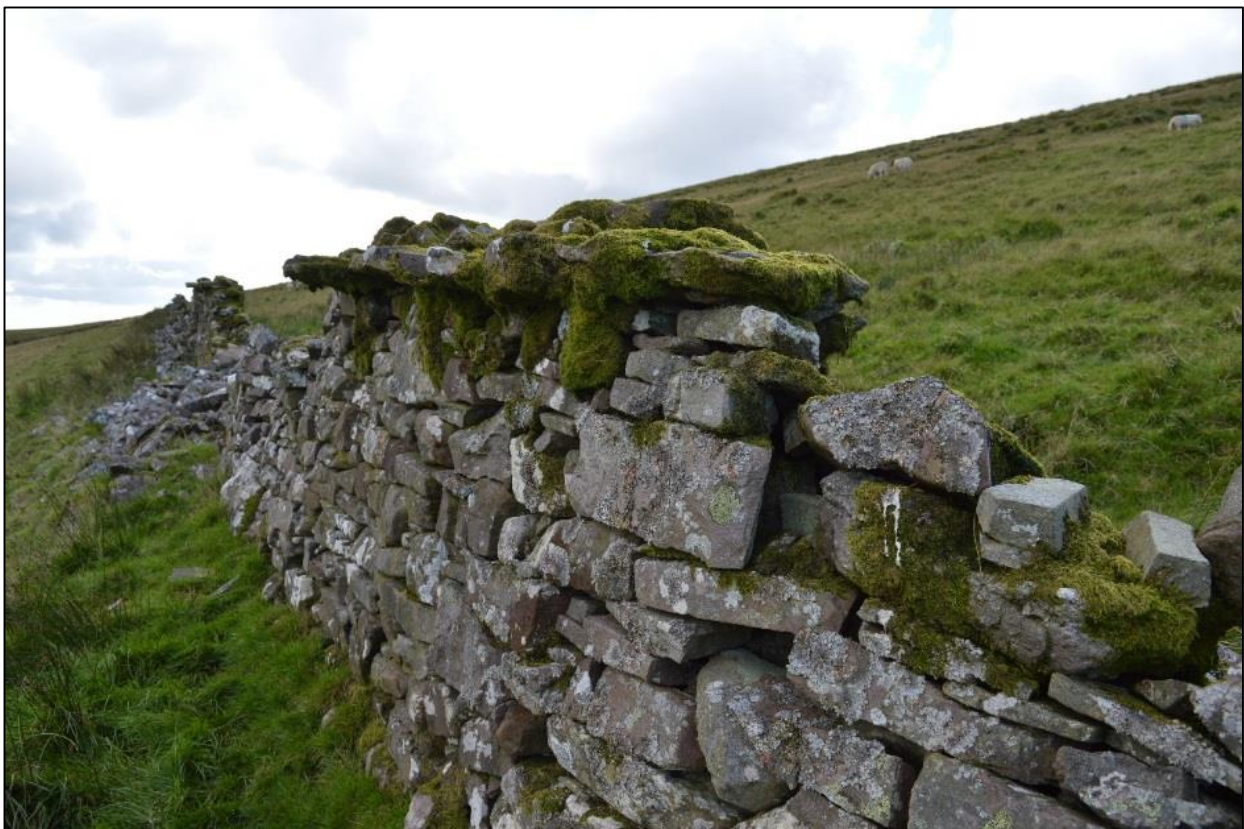
Fig. 12: Overhanging wall capping in the largest enclosure of Crai. This style of walling is found at all of the rabbit farms. Photo 4066-0004.
