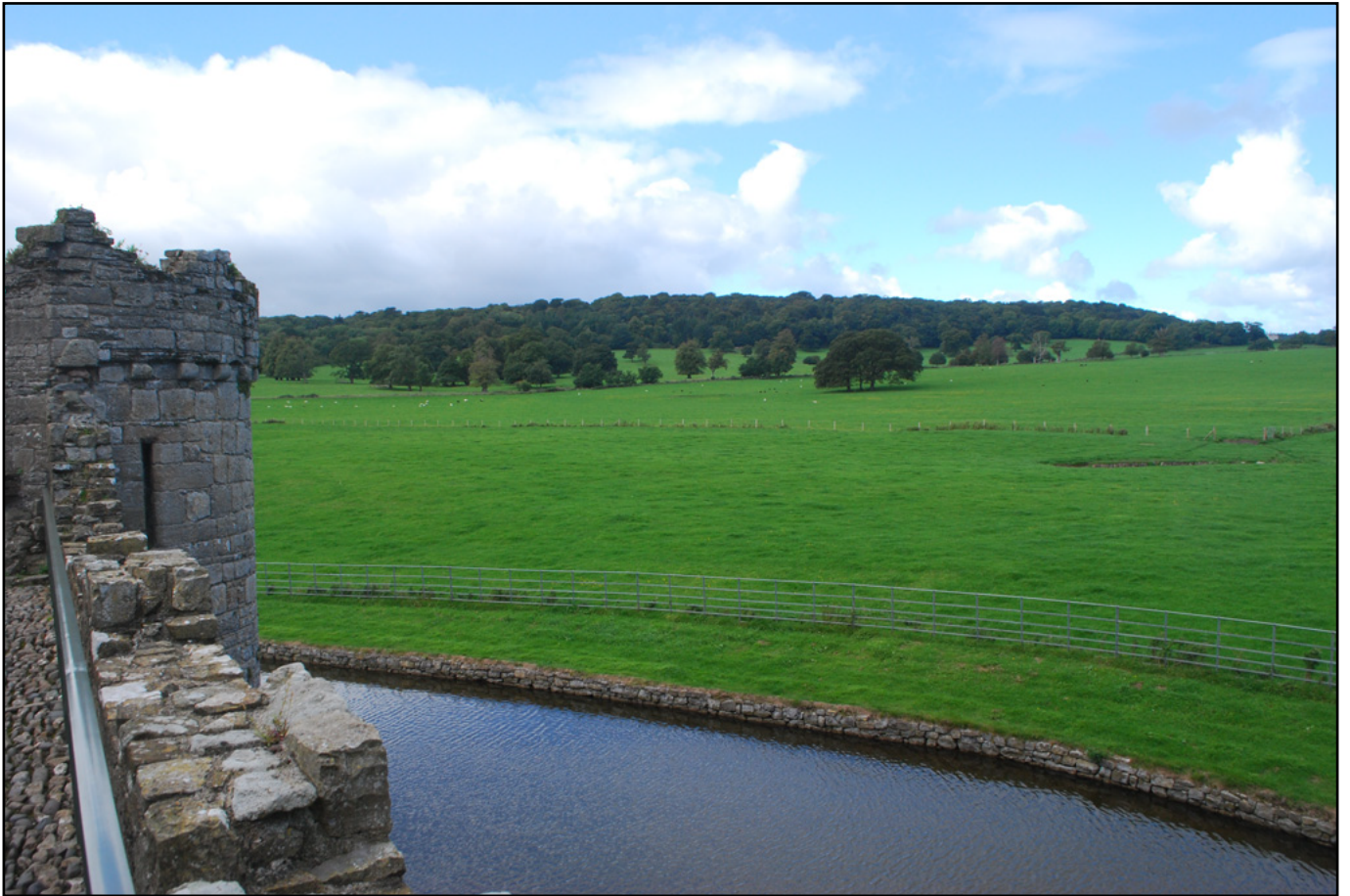
Plate 07 - View across the meadow to the north ofg Beaumaris castle from the outer curtain wall (Area 2), looking towards Baron Hill
