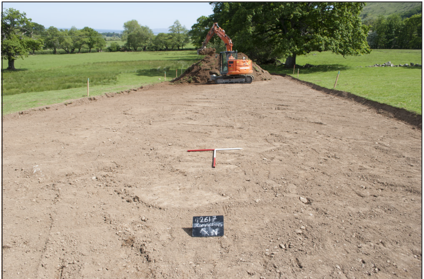
Plate 11: Shot of proposed track to Wig Farm after turf and topsoil removal; Shot from NE - scale: 2x1m (archive reference: G2617_011).
