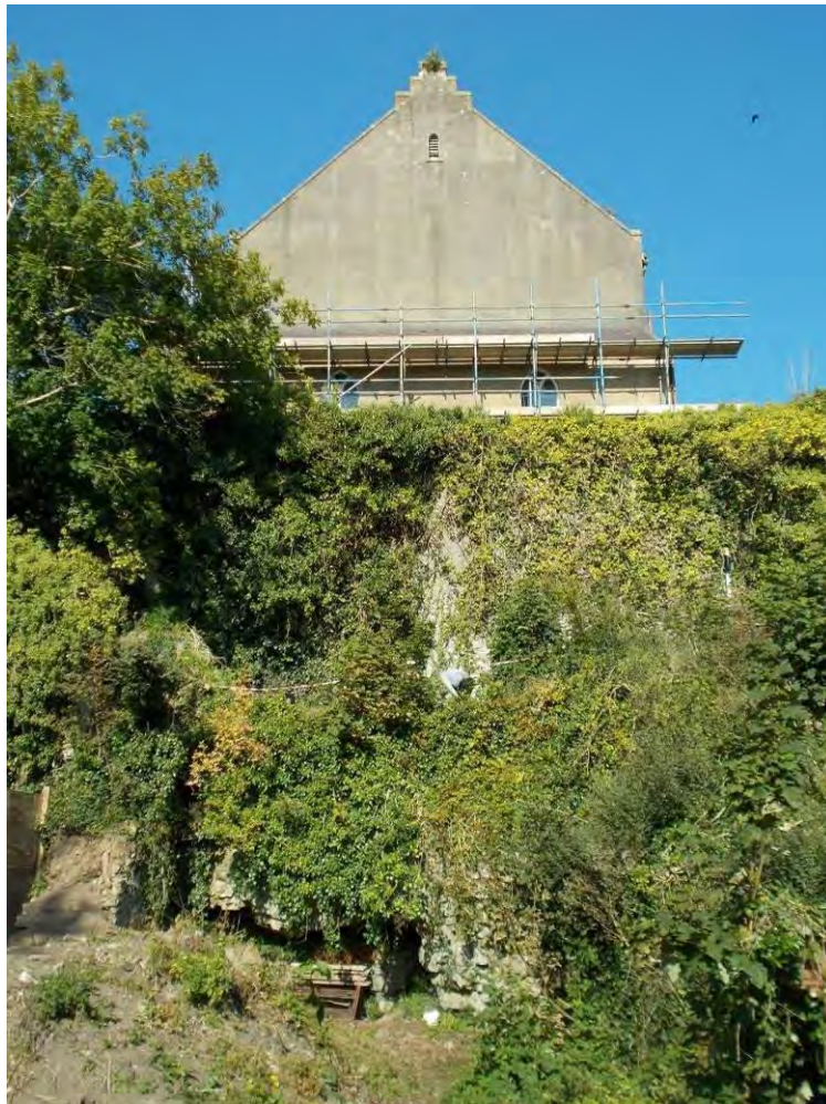
Photo 2: North facing shot of the site showing level difference between the lower eastern half, raised northern ledge, and level of the Tabernacle church to the rear.
