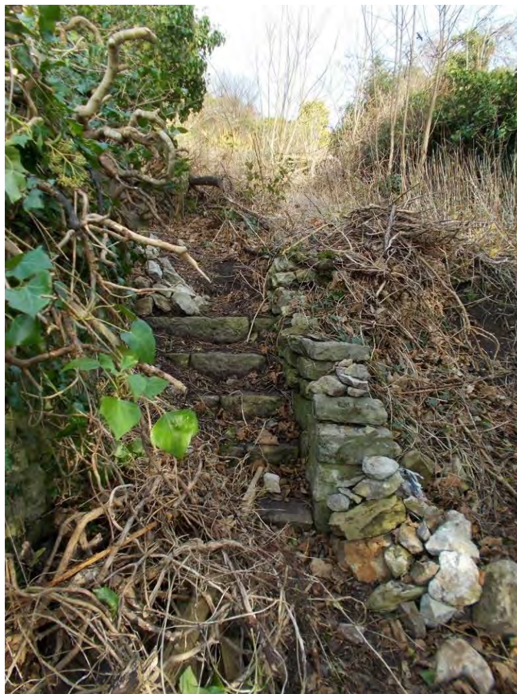
Photo 28: Steps revealed in neighbouring plot taking footpath between garden terraced against the boundary wall.
