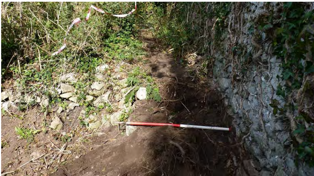
Photo 26: North facing shot of the northern-most garden terrace wall on the eastern part of the site, revealed during tree clearance work, showing the footpath along the face of the boundary wall. 1m scale.
