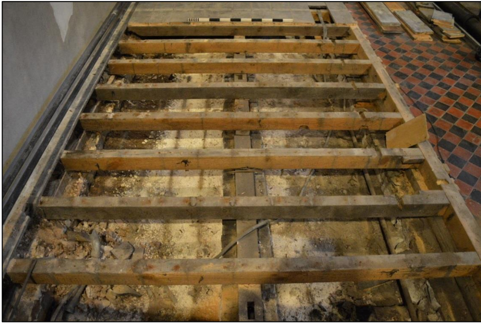
Fig. 5: The structure below the pews, showing the presumed earlier floor of the church between the sleeper walls and the north wall of the church. CPAT 4283-0009
