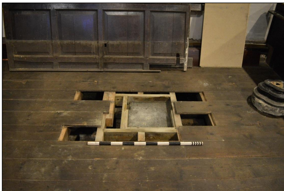
Fig. 2: The new supporting structure for the font, from the north. CPAT 4283-0001
