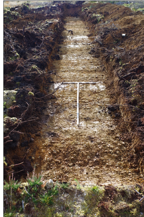
Plate 2: Trench 2, viewed from the north-east
