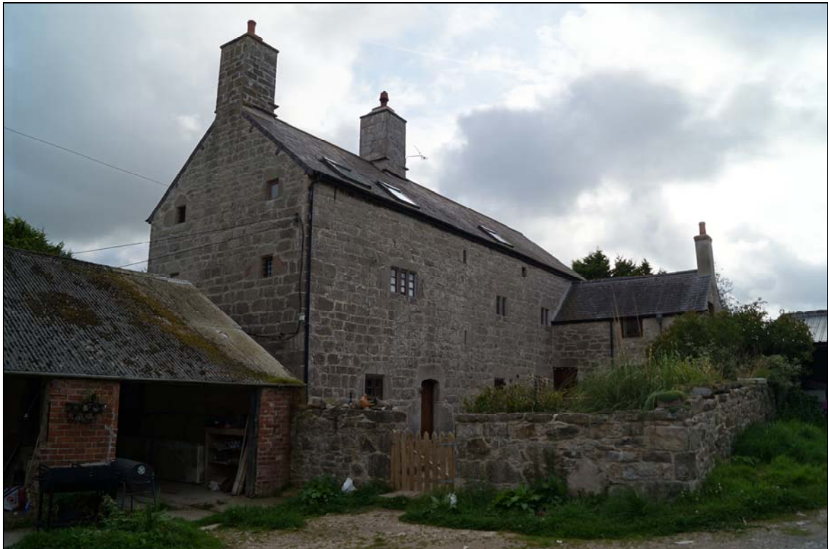
Plate 7: The substantial farmhouse (Id Number 32) looking southwest
