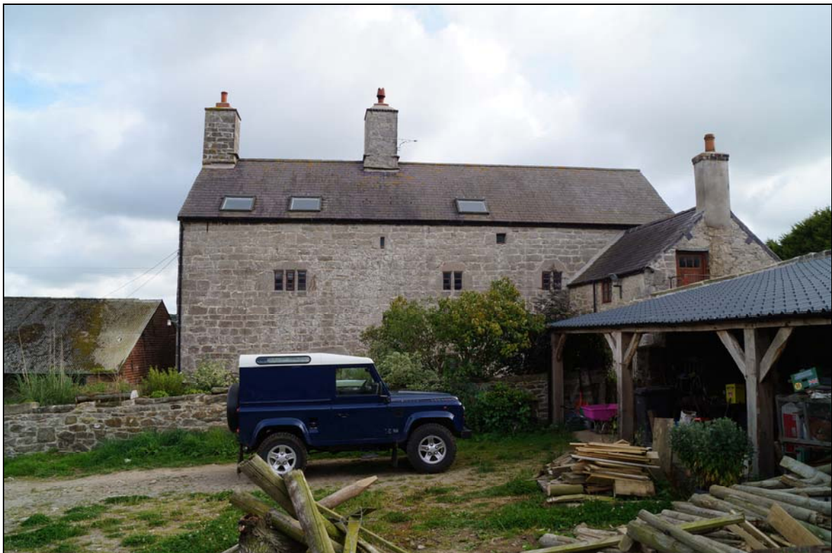
Plate 2: The northern side of the farmhouse, ID number 32, taken from the south side of the former brewhouse, ID 23, looking south across the farmyard. The proximity of this substantial house would block views of the turbine on lower ground from the farmyard
