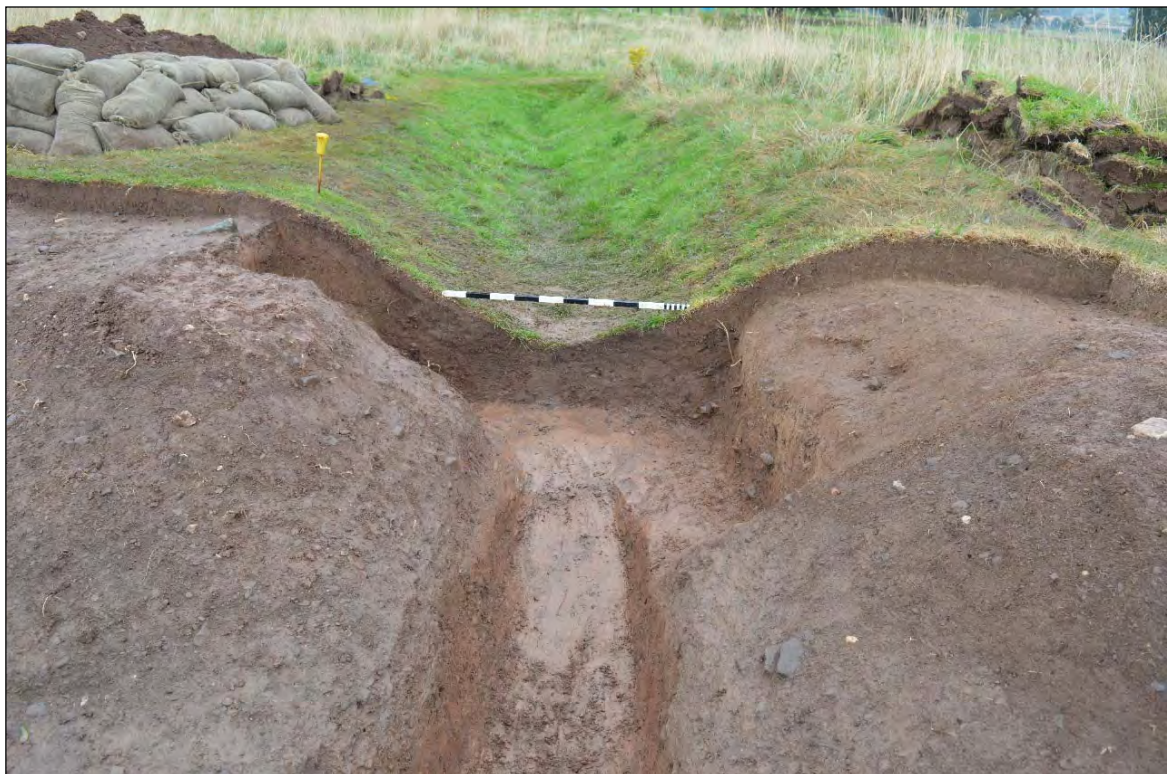
Figure 24: South-west facing section (3) through the communications trench (26). Lower section drainage duct (27) in the foreground (Photo CPAT 3916-0141).
