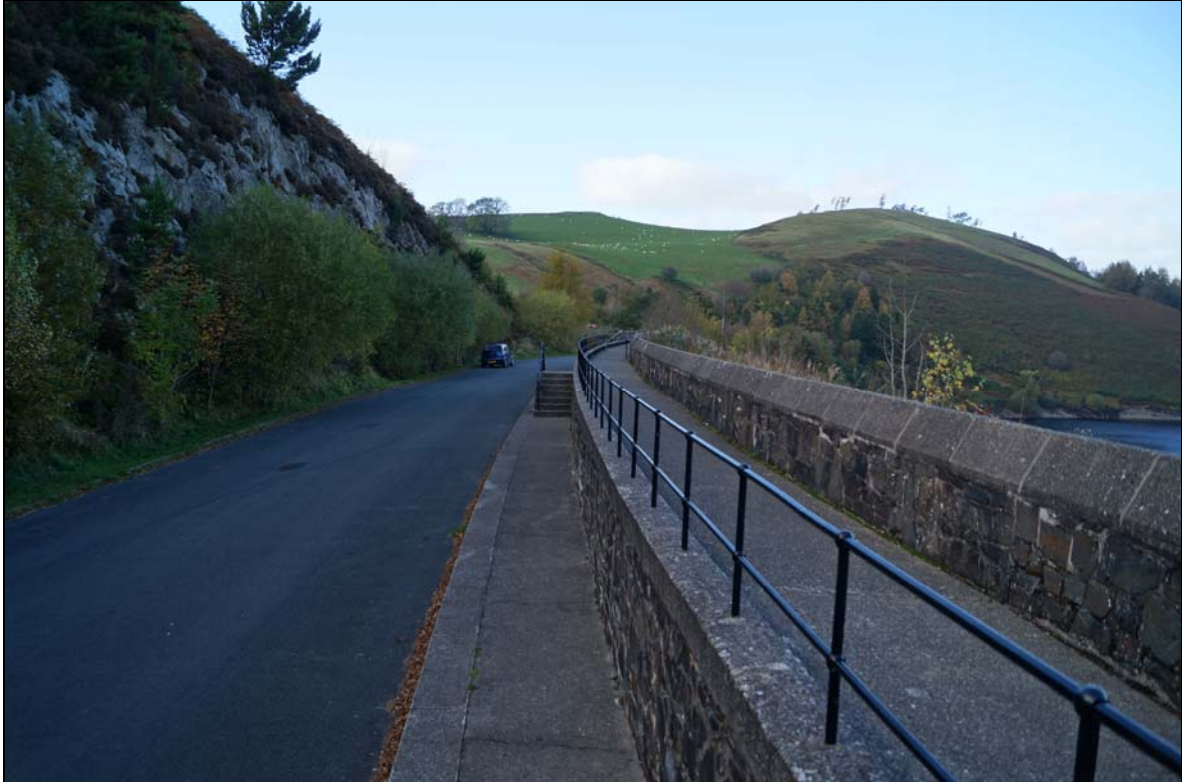
Photo 8; A view looking north-northwest along the late-20 th century concrete viewing platform at the Clywedog Dam. This feature was constructed primarily to facilitate views of the dam and the reservoir.
