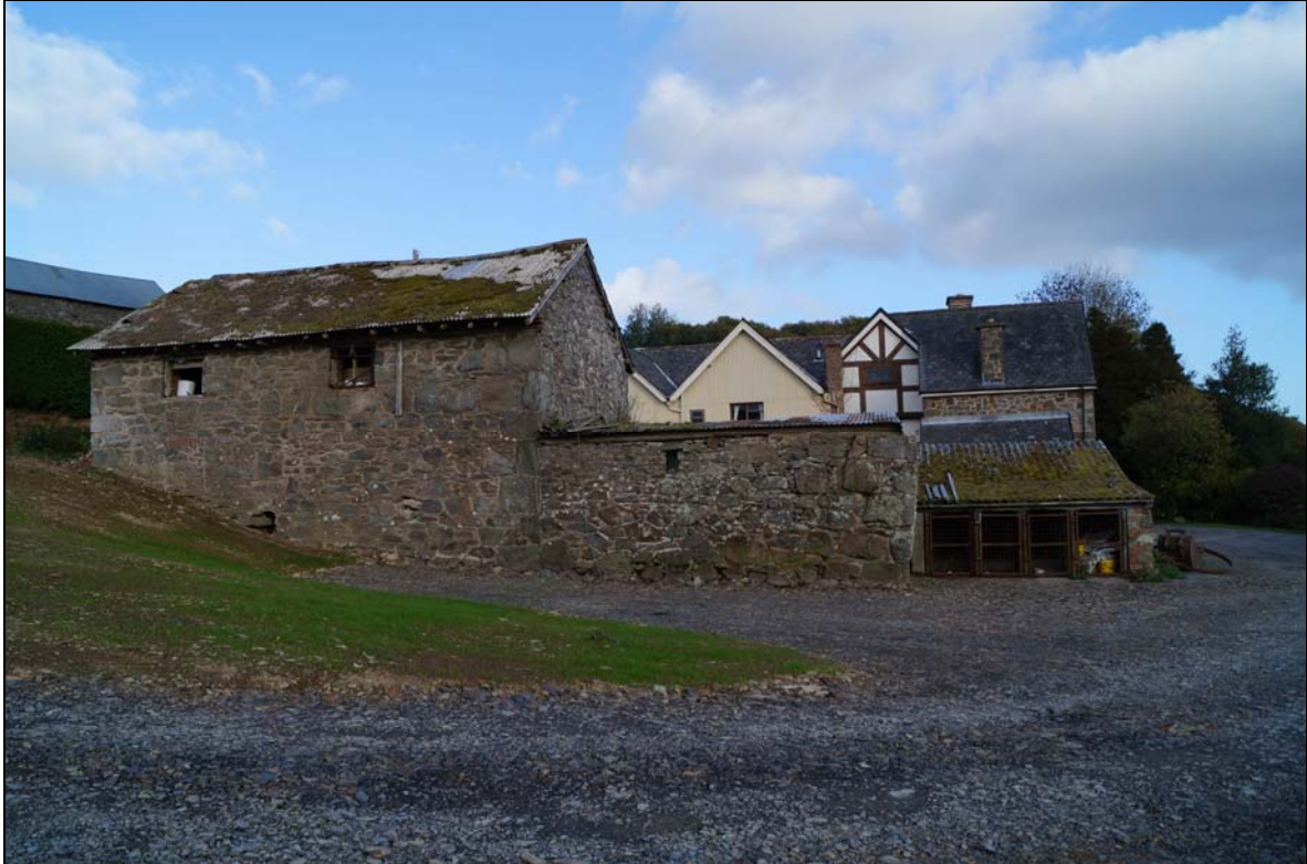
Photo 3; This view looks east towards the rear of the listed cartshed and farmhouse at Glyn. Although both buildings are visible or partly visible, the important architectural details of both, which are predominantly in their east-facing elevations, are not visible. This would not be considered to be a key view of either building. The blade tip of the proposed turbine may be visible above the treeline at the centre of this image.
