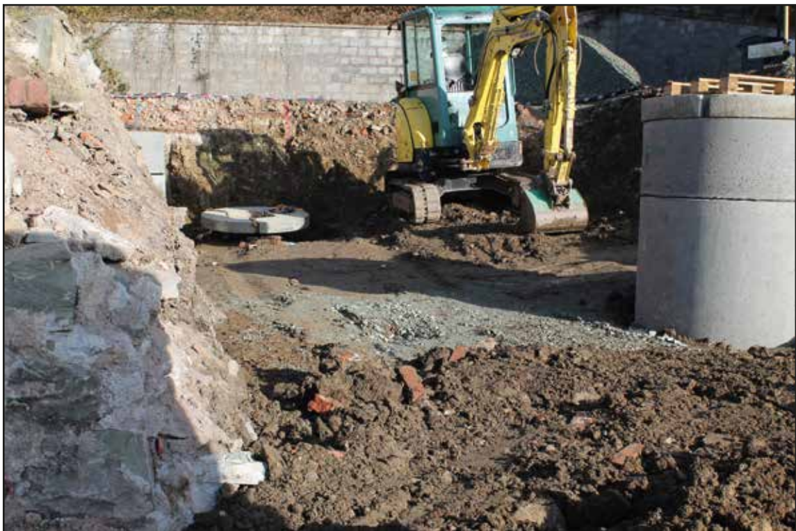
Plate 2. Area B after excavation, looking N.
