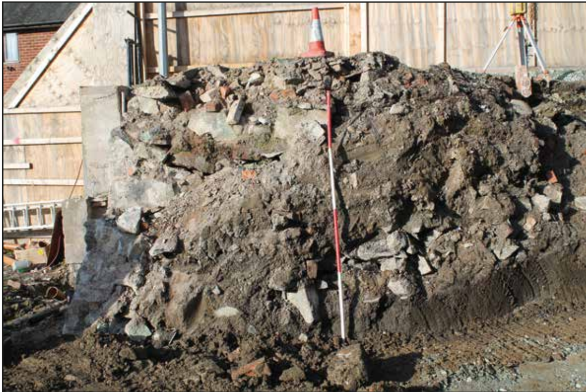
Plate 3. Area B after excavation, looking W.
