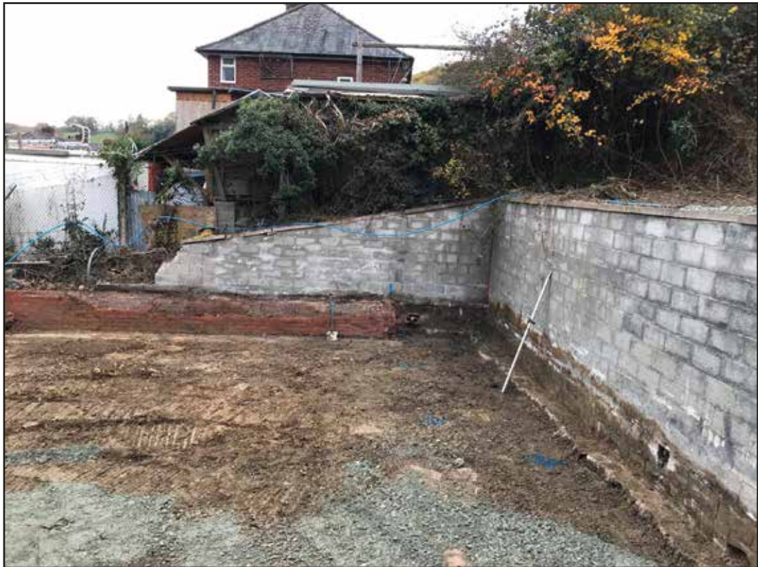
Plate 1. Area A after groundworks, looking W.
