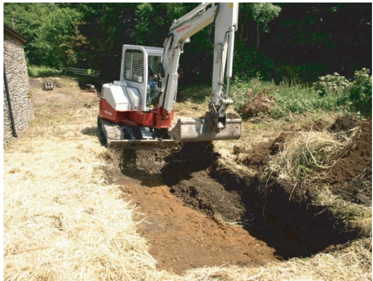
Plate 3. Working shot. Trench 3. Looking east.
