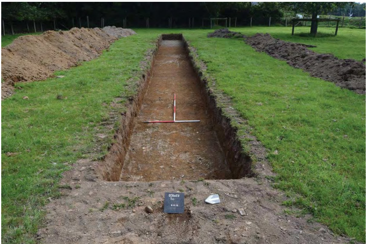
Photo 32: Trench 10, after machine excavation and initial cleaning. View Southeast. 2m & 1m scales.
