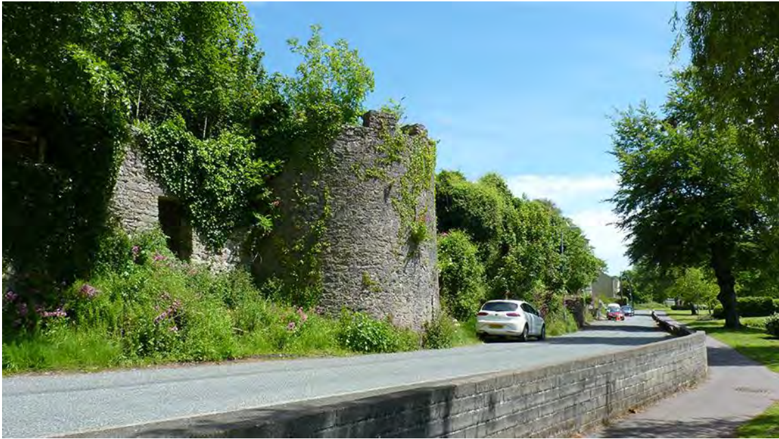
Photo 3: View ESE along Common Road at the Gun tower (SAM PE015, LB 6342)
