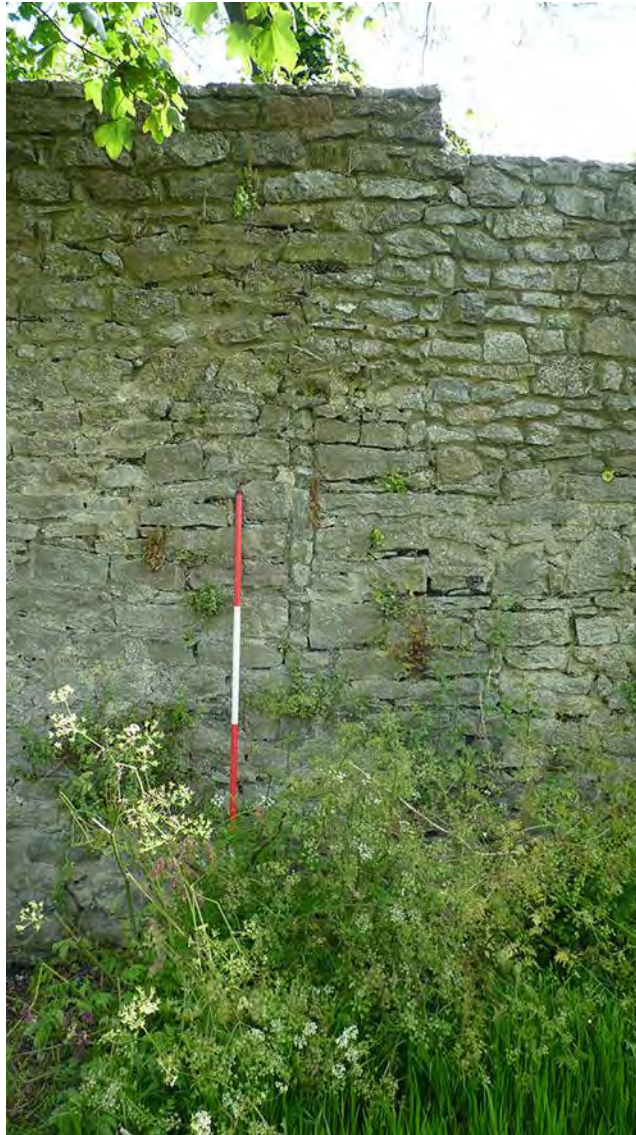
Photo 7: An infilled arrow loop within the town wall (LB 6342) between the site and the gun tower, believed to be evidence of the medieval origin of this section of wall. 2m scale.
