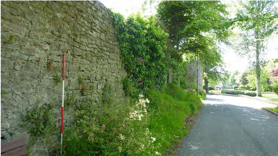
Photo 8: View ESE from the blocked arrow loop (immediately to the right of the scale) towards the Gun Tower. 2m scale.
