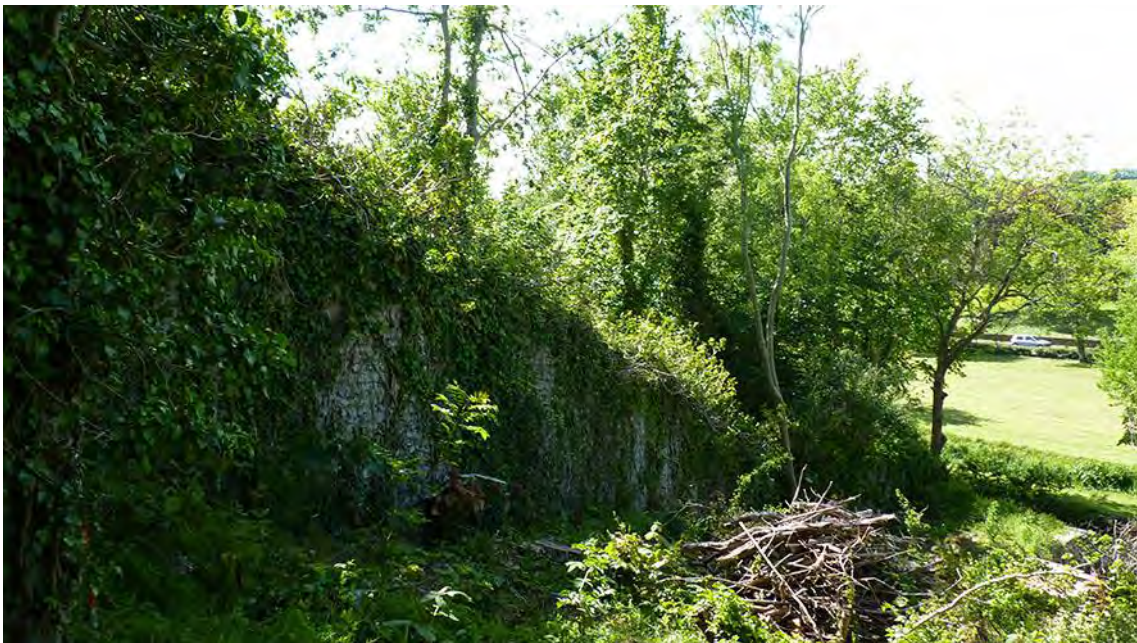
Photo 15: View SSE down the eastern boundary wall.
