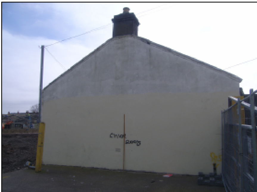
Plate 2 Cottage north elevation
