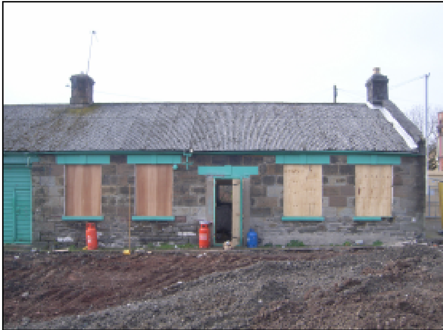
Plate 1 Cottage façade (east elevation)
