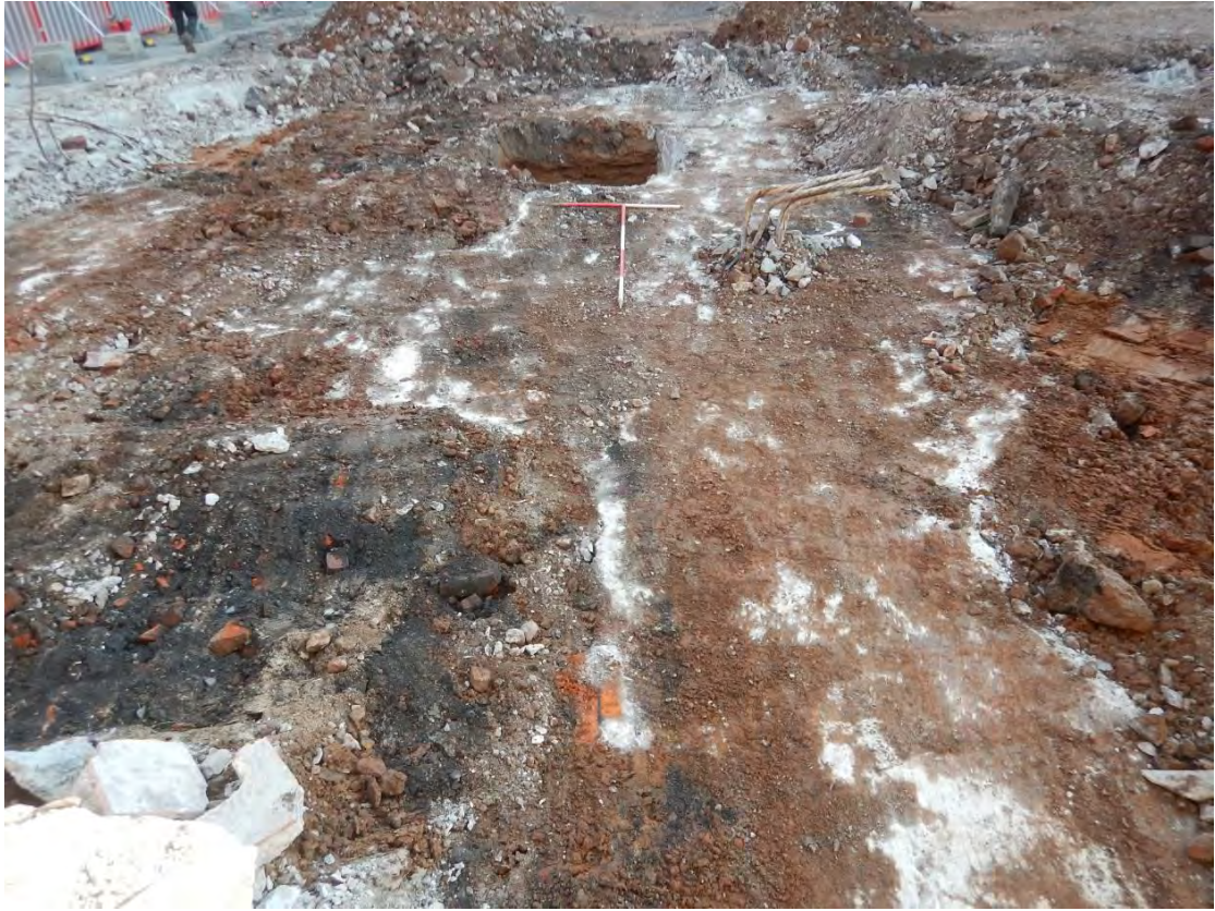
Photo 13: Concrete foundations 020, view facing south. 1m & 2m scales.
