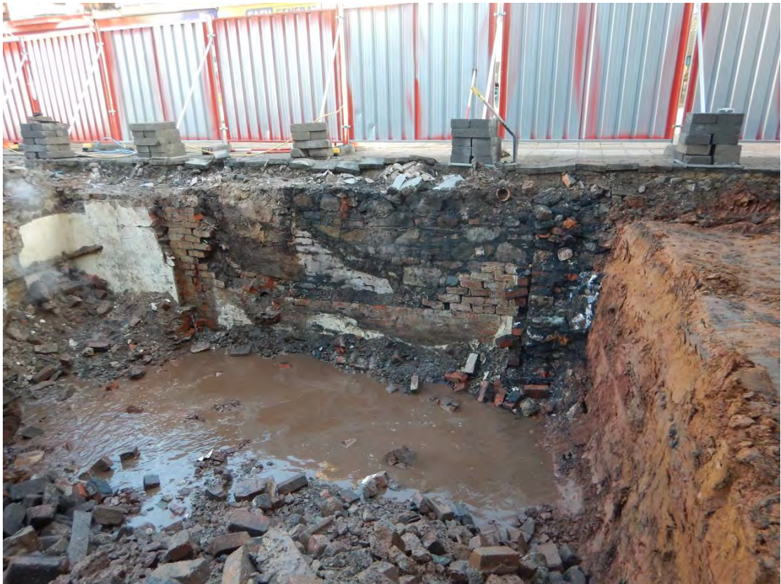
Photo 6: Stone wall 012 revealed behind brick-built cellar wall 005. View facing northeast.
