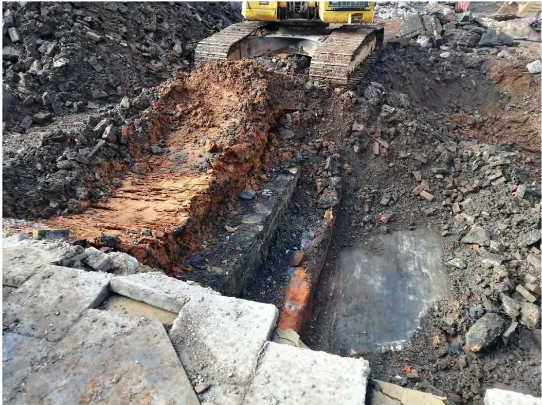
Photo 15: Cellar 026 during excavation, view facing southwest.
