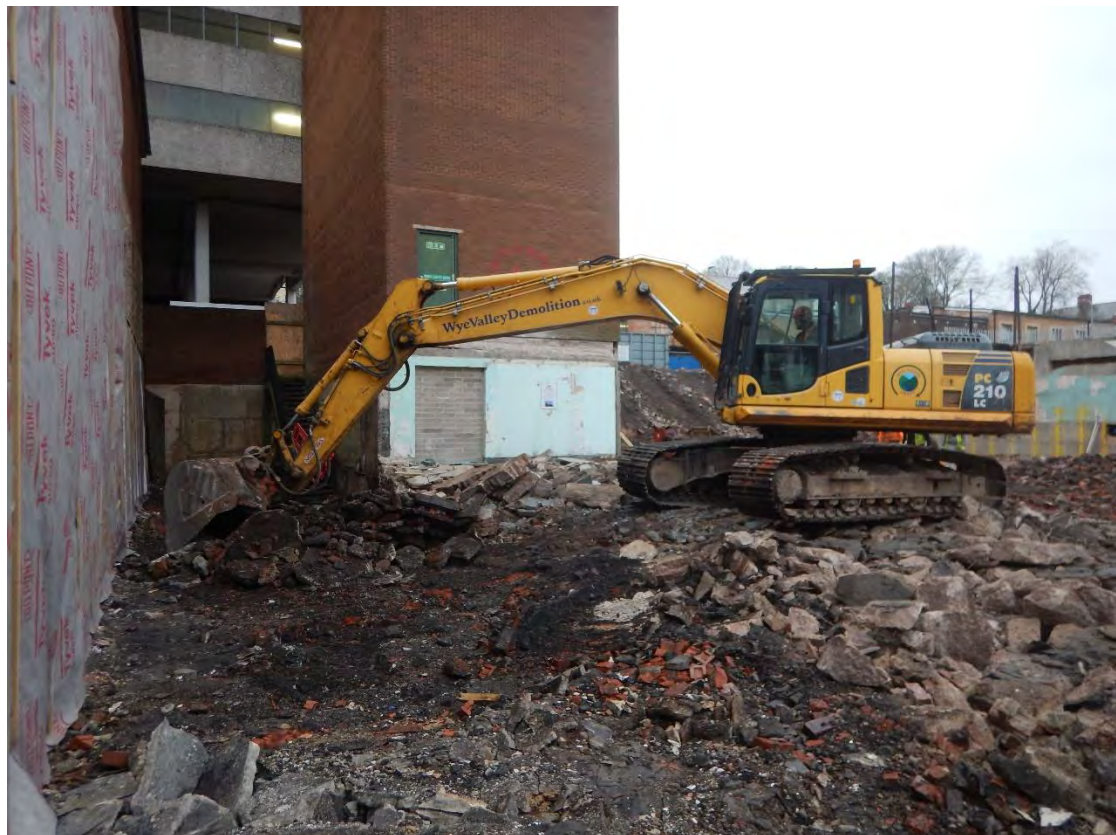
Photo 2: As above, view facing SW.
