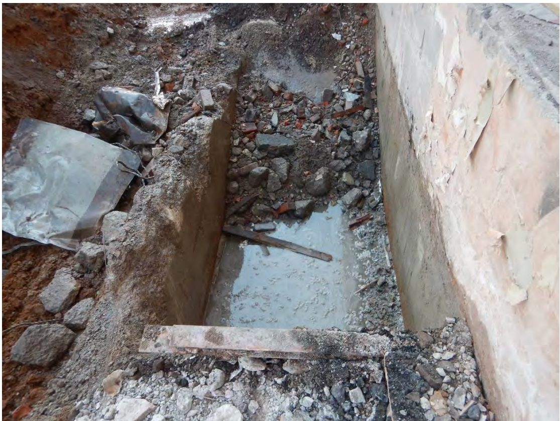
Photo 12: Escalator sump 016, view facing west.
